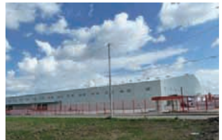
NEW PLANT IN PUEBLA, MEXICO; INTERIOR AND EXTERIOR MODULES
