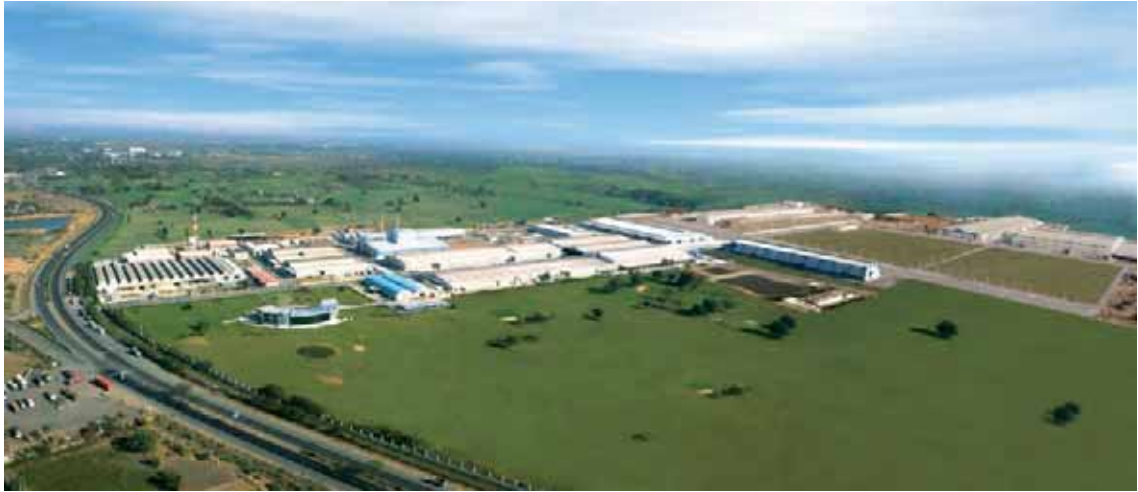
Kemrock manufacturing facility in Asoj, Vadodara
