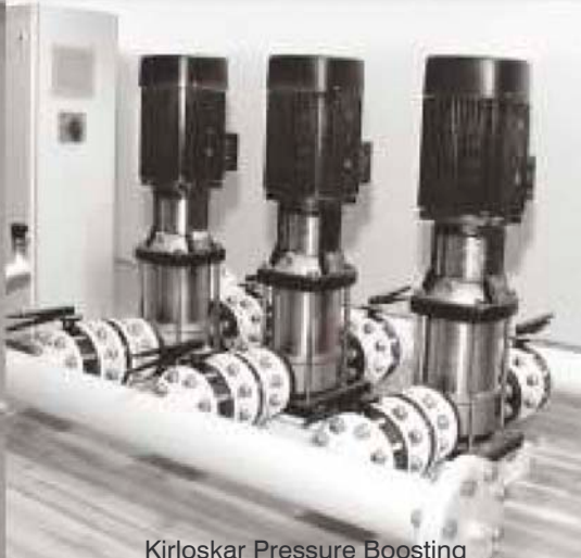
Kirloskar Pressure Boosting (Hydro Pneumatic) System
