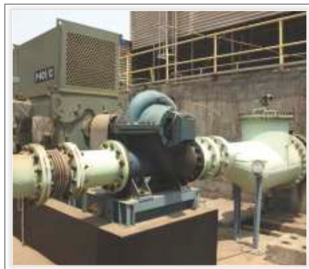
LLC pump installation at National Peroxide Limited, Kalyan
