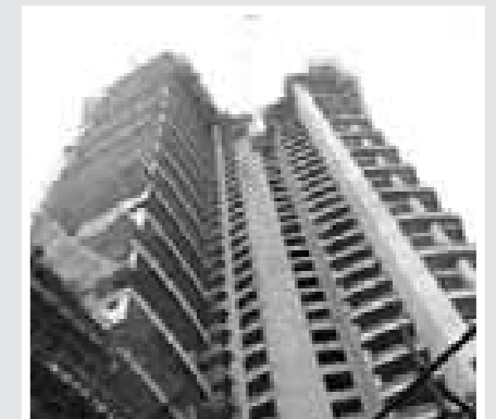
Construction of 64 Storied Residential Sale Tower at Mumbai
