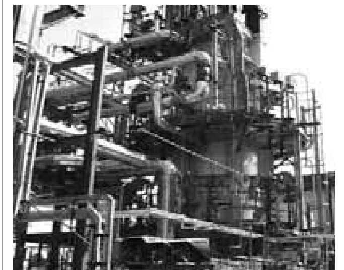
Piping and Equipment installation for MSQ Project IOCL Refinery, Digboi, Assam
