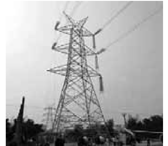
Construction of 400KV D/C QUAD Transmission Line from Siliguri to Bongaigaon
