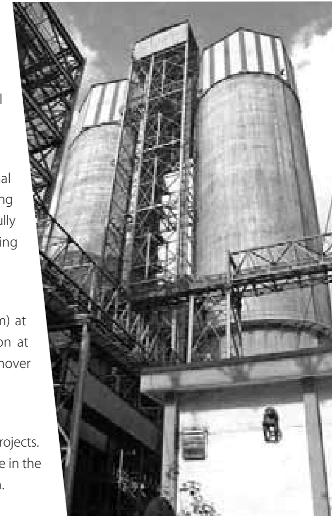
Construction of 66 M high Cement Silo for ACC Cement, Chandrapur, Chhattisgarh
