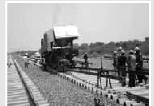
Imported flash – butt Welding Machine working for a track doubling project in A.P. for RVNL
