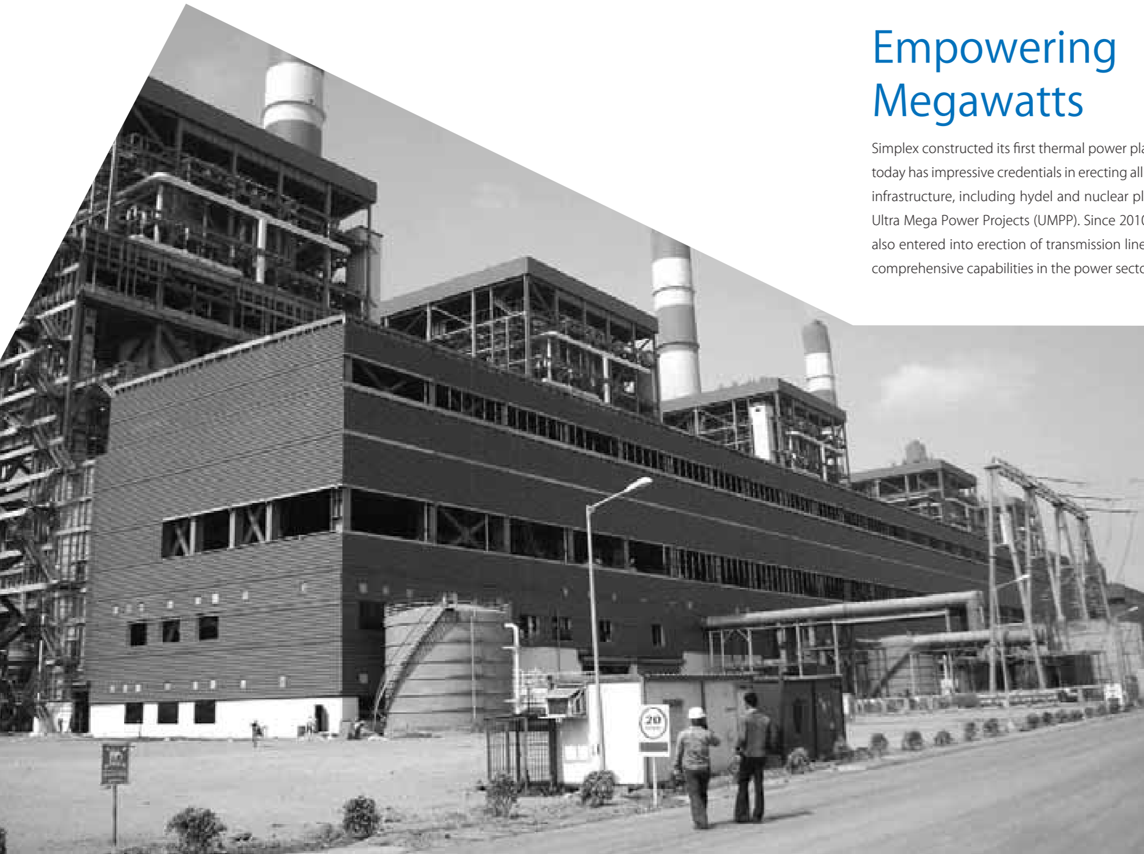
5 X 800 MW Ultra Mega Power Plant of Tata Power at Mundra, Gujarat
