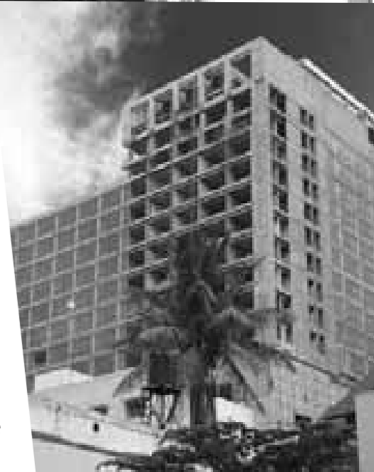
Construction of Ritz Carlton Hotel, Bangalore
