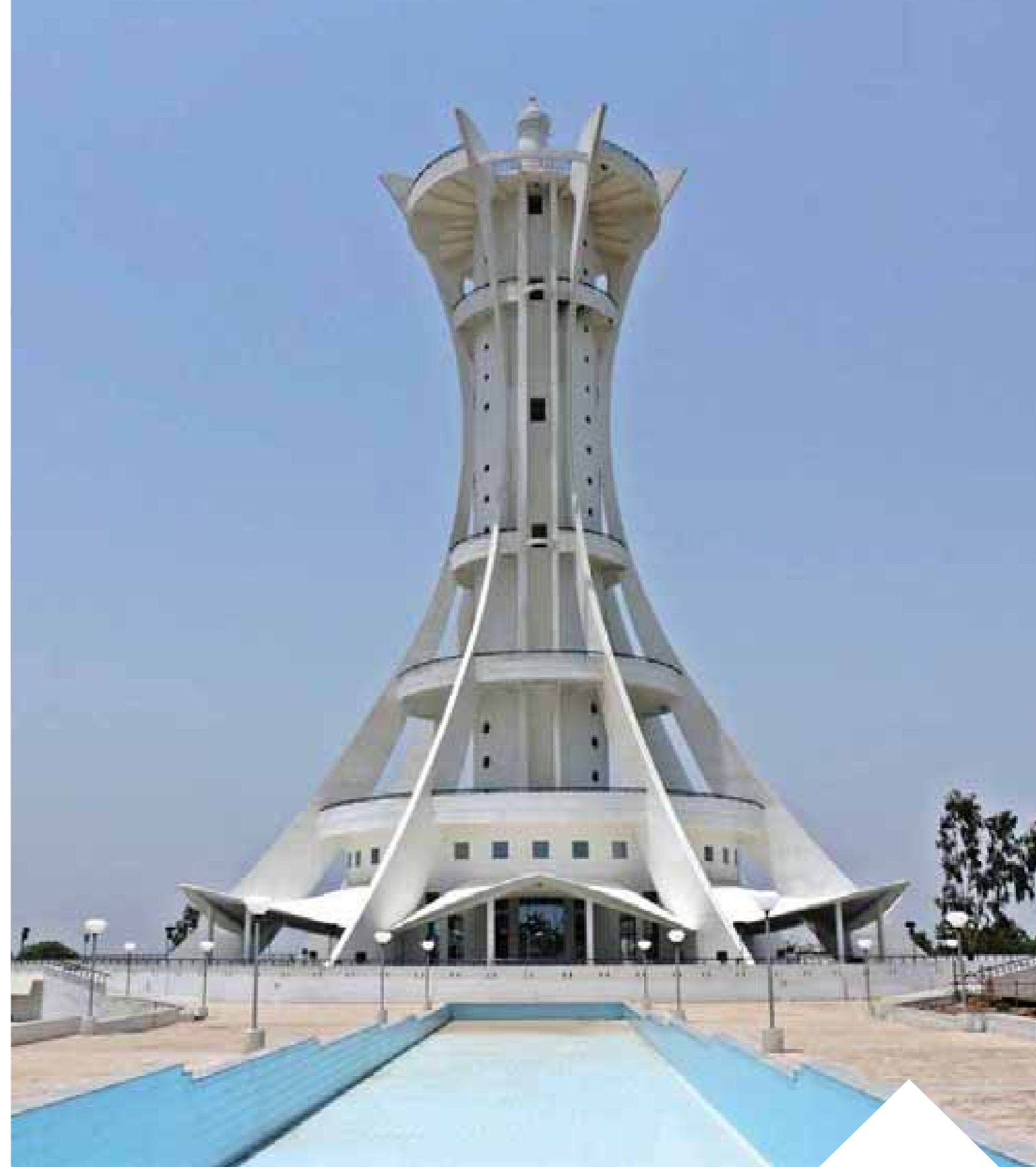
Construction of 77M high Jaikhamb Tower at Girodpuri, Chhattisgarh
