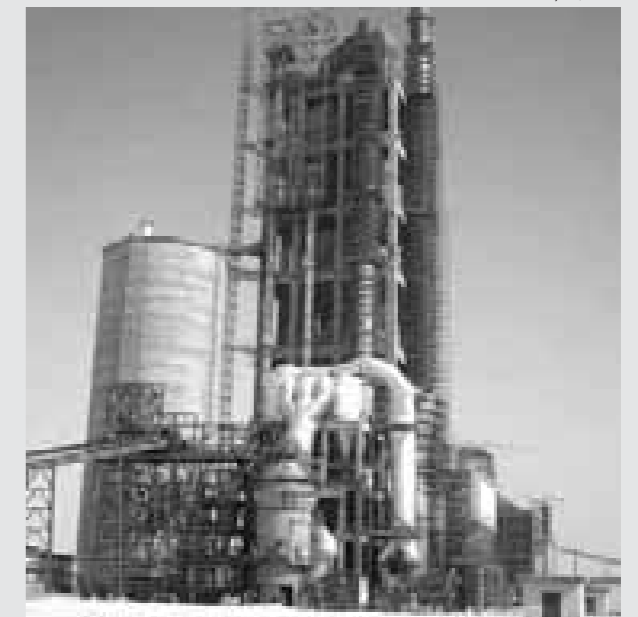
Cement Plant - UMM - BAB at Doha, Qatar
