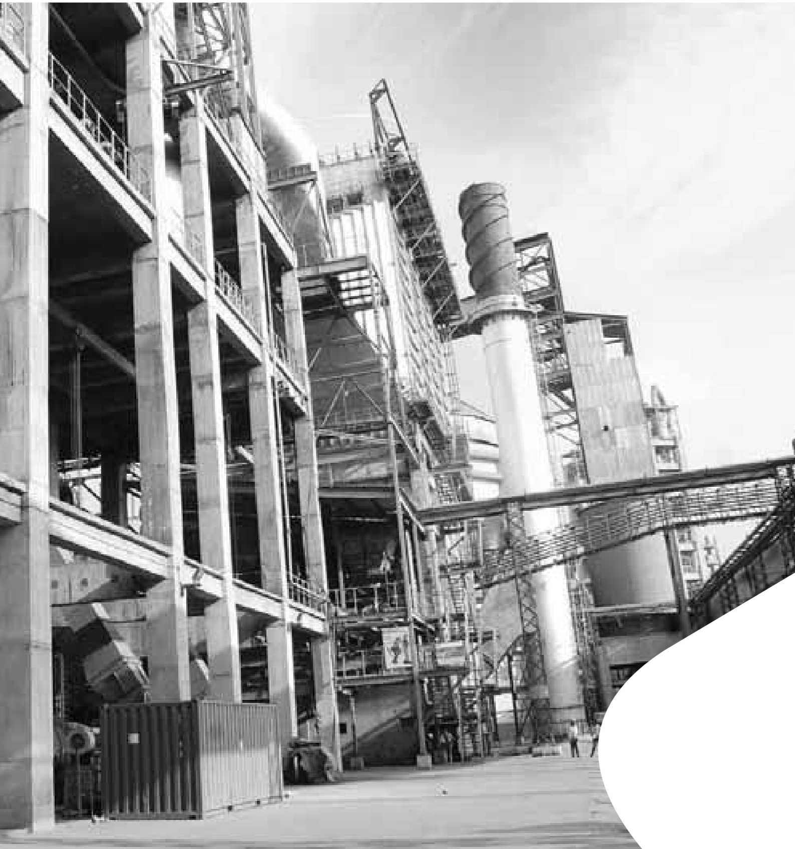
A view of Coal Mill Building for ACC Cement at Chandrapur, Chhattisgarh
