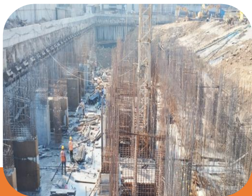
Foundation Work Completed Basement – 3 rd Slab RCC completed
