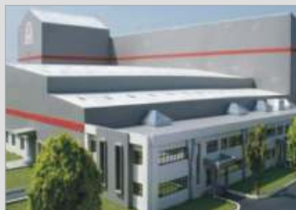
New Power Transformer, Distribution Transformer & Medium Voltage Switchgear Unit at Vadodara
