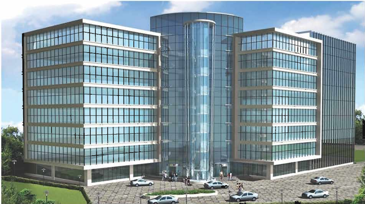
Commercial Complex, IT Park, Nahur, Mumbai.
