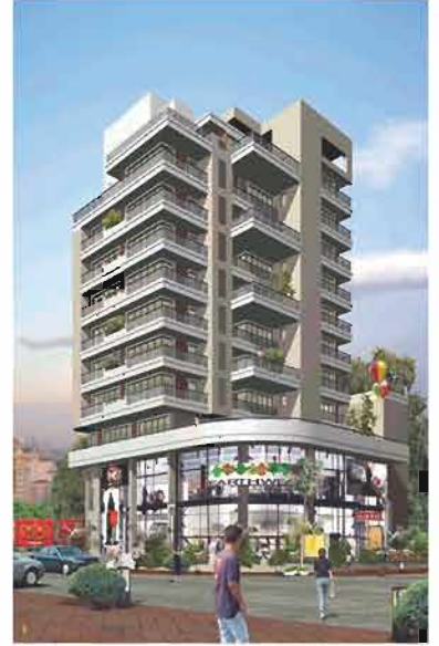
Commercial/Residential Complex, Centre Point, Bandra, Mumbai.
