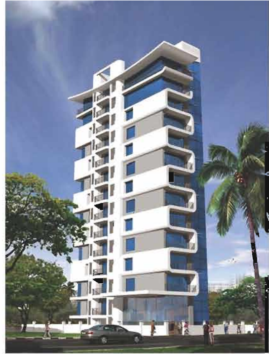
Residential Complex, Pali Naka, Bandra, Mumbai.
