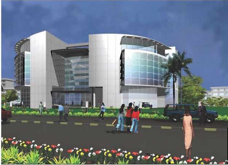
Commercial Complex, Kaledonia, Andheri, Mumbai.
