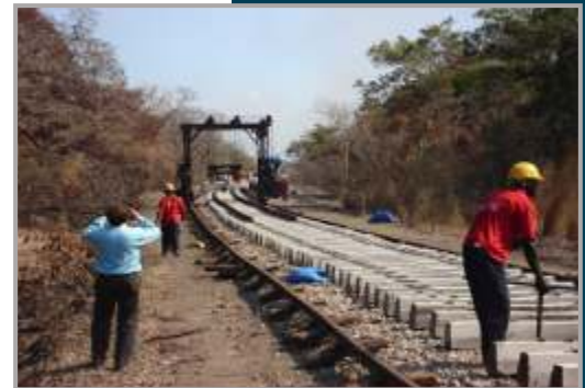
Laying of Track, Mozambique
