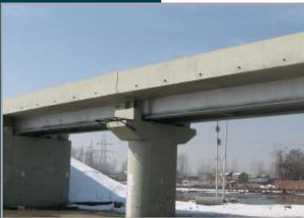
A bridge at Udhampur for New Railway Line Project (Jammu & Kashmir)
