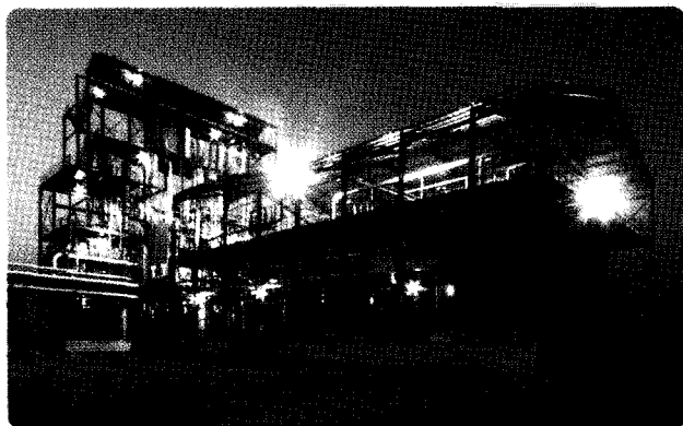
Brijnathpur ethanol plant commissioned in 2008
