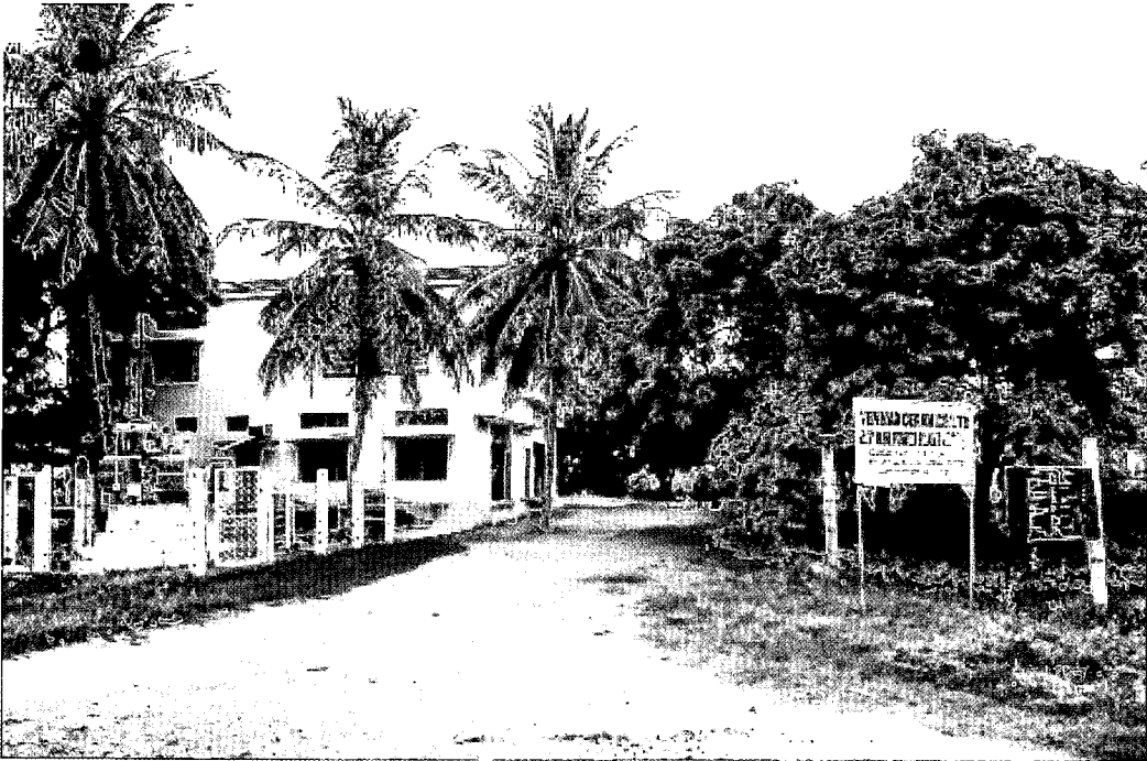
Vennar Ceramics Limited (Power Plant)
