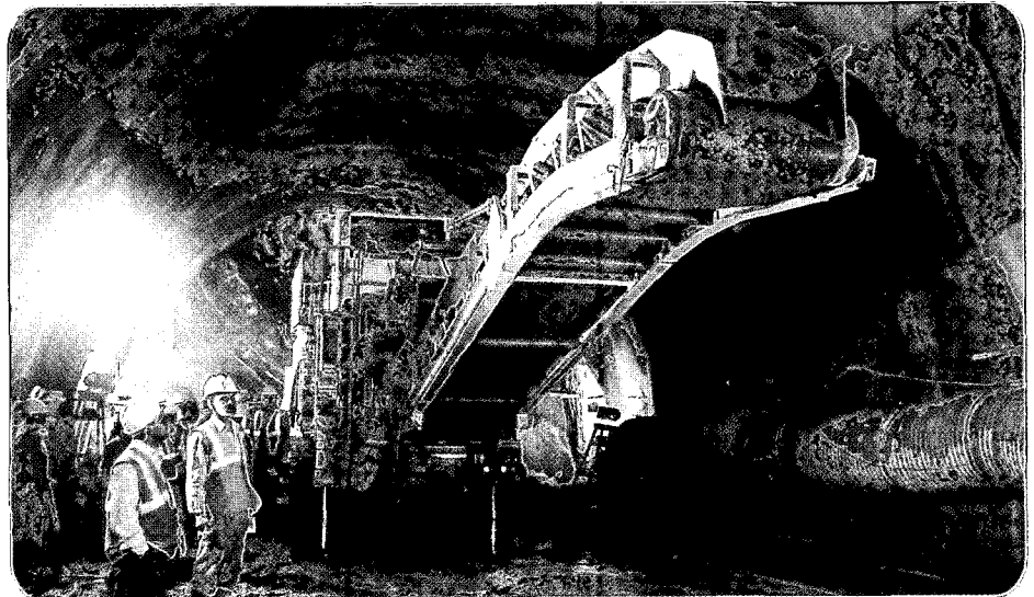
T-80 Tunnel - J&K Project
