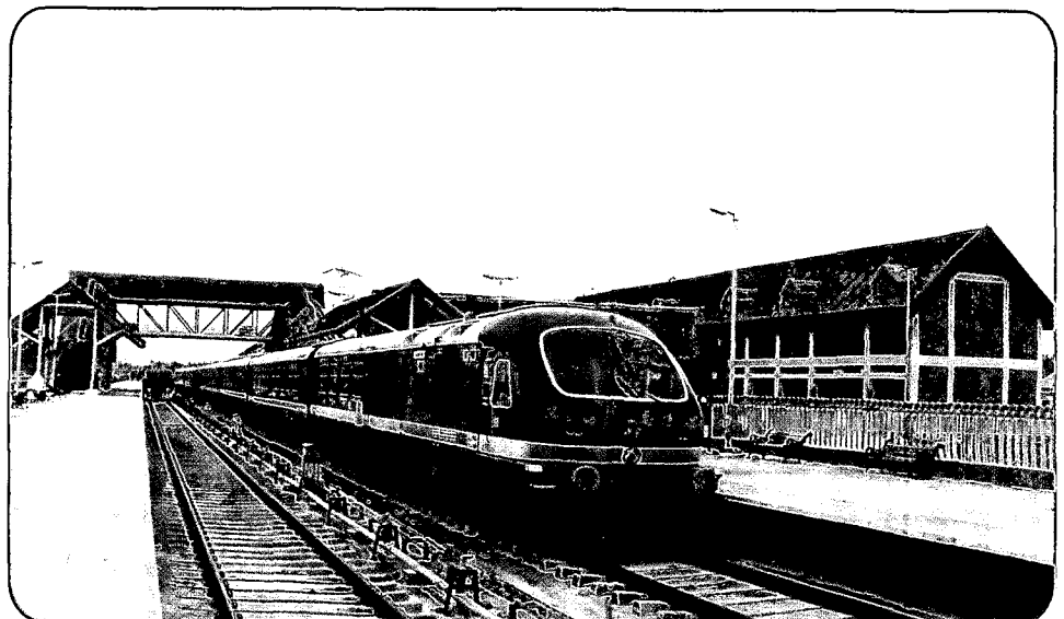
Completed View of Budgam Railway Station - J&K Project
