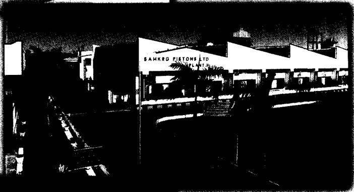
Varisam - Rings Plant (Near Visakhapatnam)
