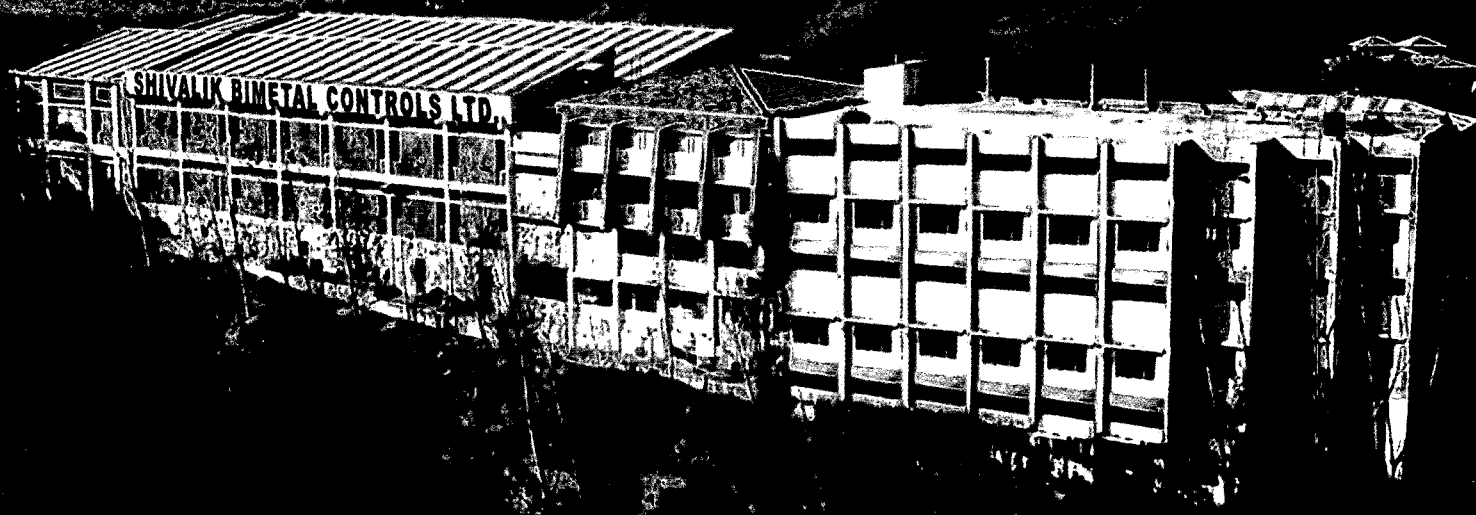
SBCL Plant at Chambaghat, Solan, Himachal Pradesh
