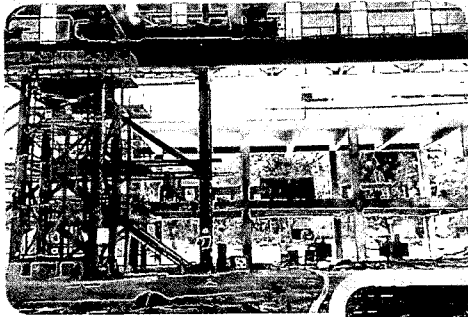
Induction Hardening Equipment under Erection
