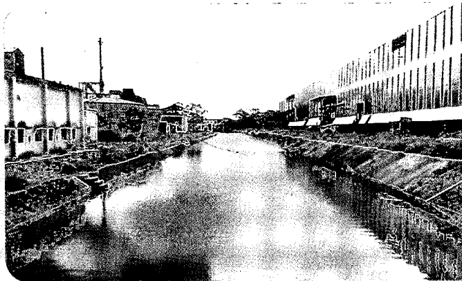
Rain Water Harvesting
