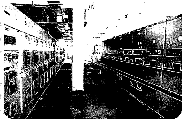
Main receiving Sub-Station
