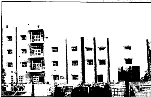
Manufacturing Facilities (Unit-3)
