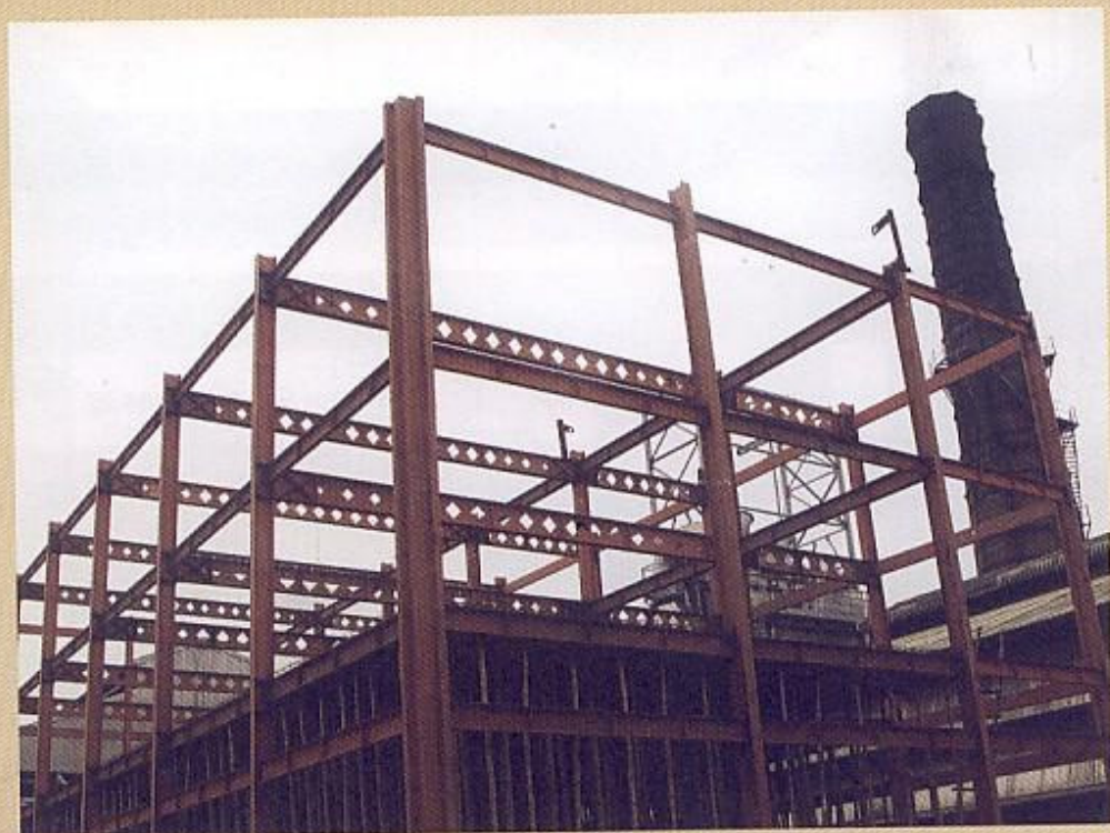
▲ New industrial building under construction
