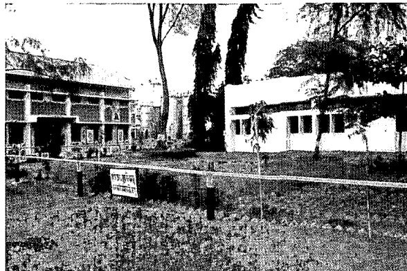
View from Inside Gate
