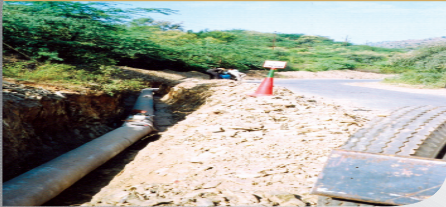
Cross Country Pipeline
