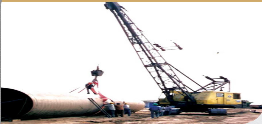
Large Diameter C.W. Piping Work for Power Plant
