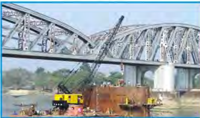
Jubilee Rail Bridge across River Hooghly, West Bengal
