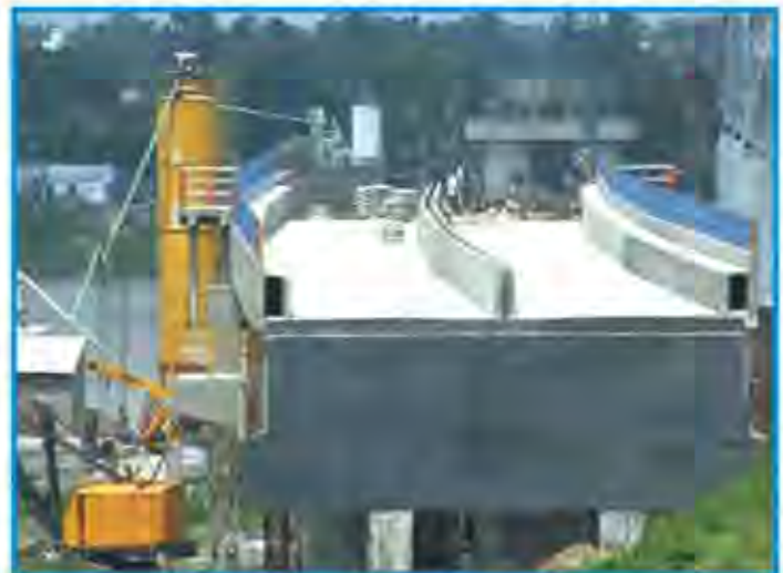
View of Nainital Side Viaduct (4 Spans)
