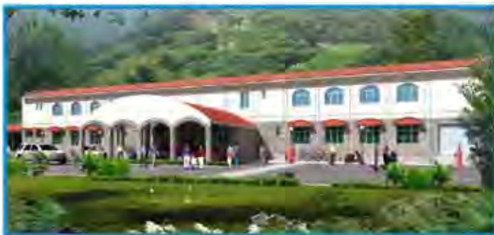
Reasi Station Building Jammu & Kashmir
