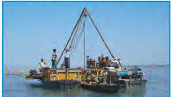
Under water sub-surface investigations rail-cum-road bridge on River Brahmaputra
