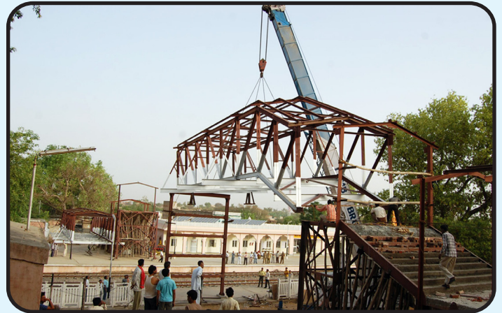
Launching of FOB across four tracks in Rewari - Fulera Station
