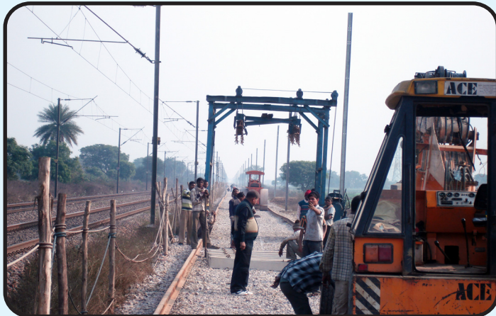
Laying of Sleeper in third line of Aligarh - Ghaziabad Section
