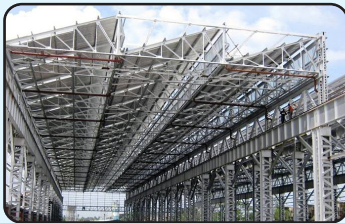
Construction of Dhankuni workshop shed (Front view)
