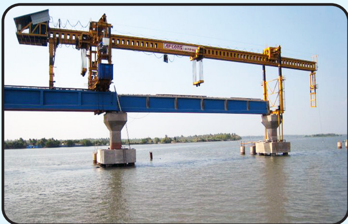
Launching of girders in Idapally - Vallarpadam Bridge on backwater in Kochin
