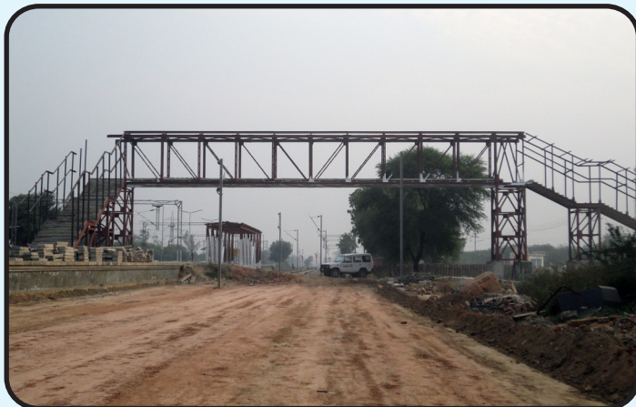
Formation work for third line in Aligarh - Ghaziabad Section
