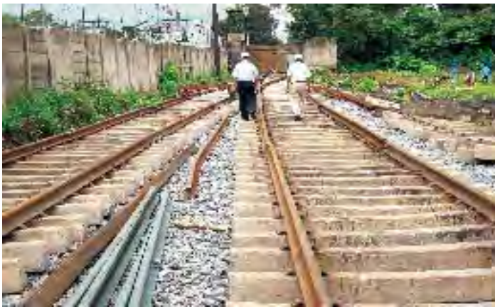
Restoration of Railway Siding inside the premise
