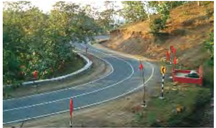
Road in Hill Section, Narsinghpur-Harrai-Amarwara Road Section, NH-26B, Madhya Pradesh
