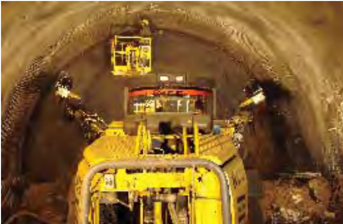
Construction of Pirpanjal Tunnel in progress near Banihal in J & K
