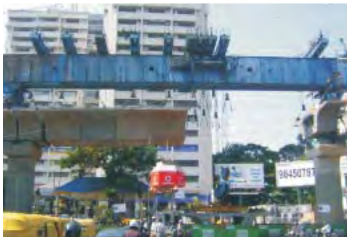
Bangalore Metro - Erection of precast segment of viaduct in progress
