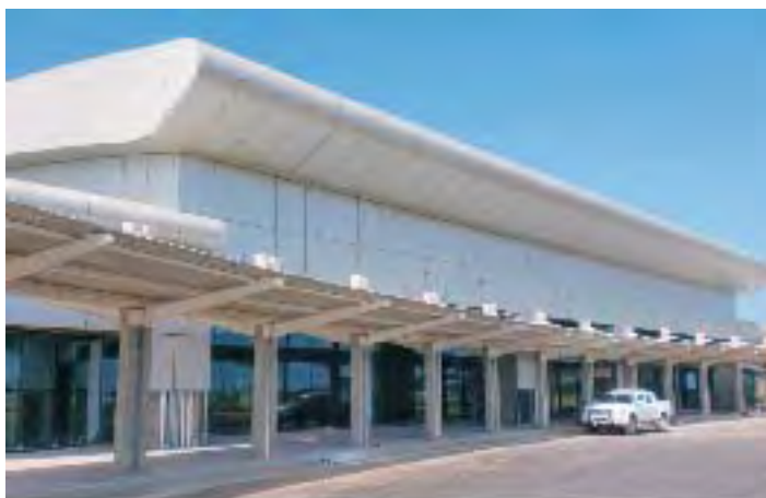
Main Entrance of Terminal Building at Francistown Airport, Botswana
