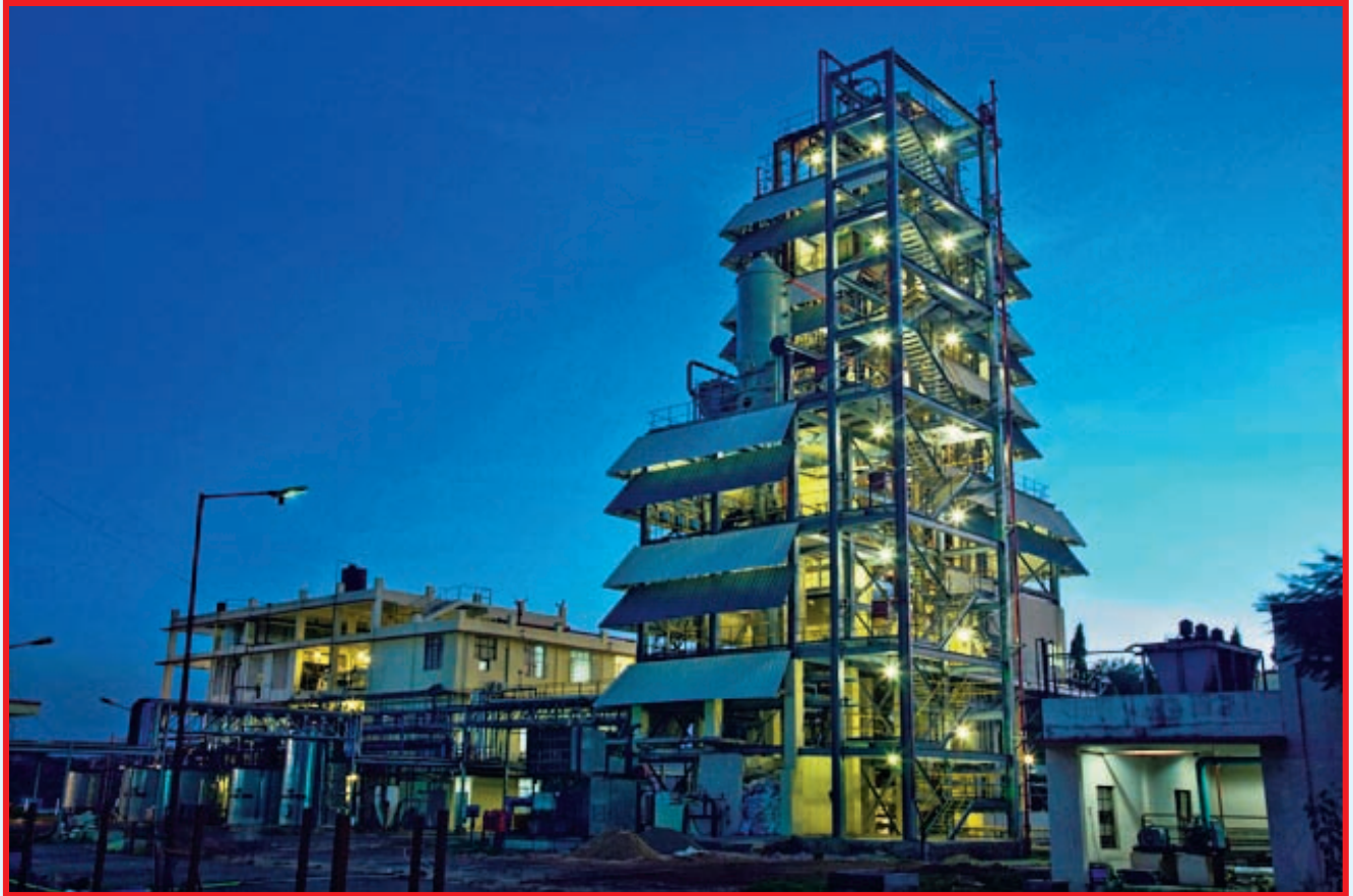
A View of the EPS Plant near Chennai
