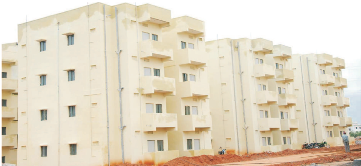
GHMC (BSUP) Project, JNNURM, Hyderabad, Andhra Pradesh
