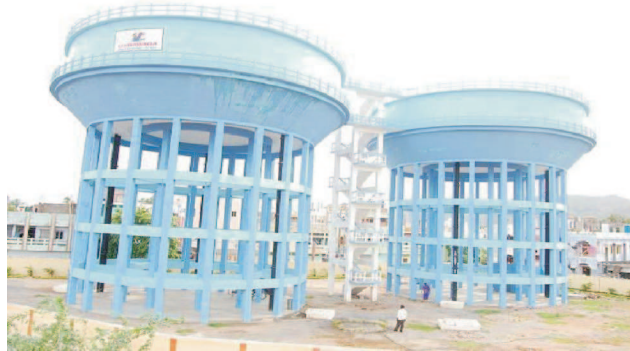
Water Tank, Vijayawada Project, JNNURM, Hyderabad, Andhra Pradesh
