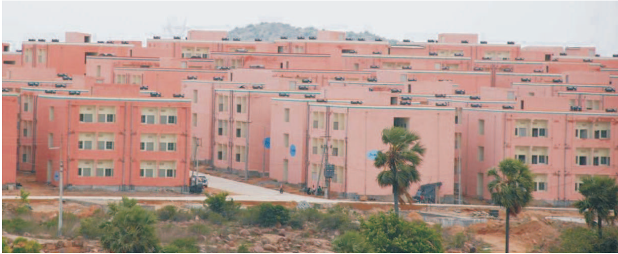
BSUP Project, Hyderabad, Andhra Pradesh
