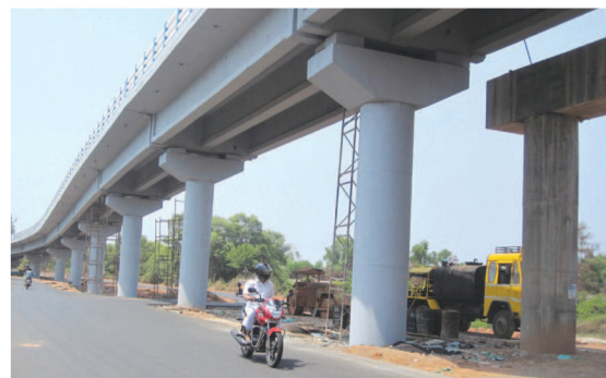
Railway overbridge (Roads & Bridge Development Corporation of Kerala)
