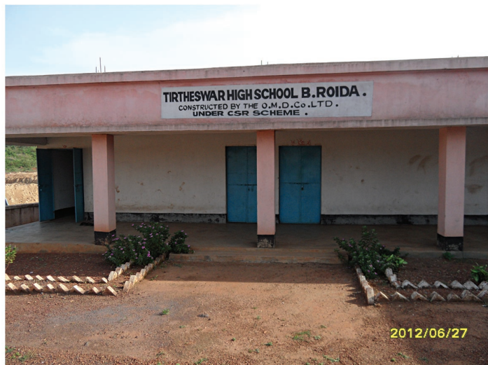
School building constructed by OMDC under CSR Scheme.
