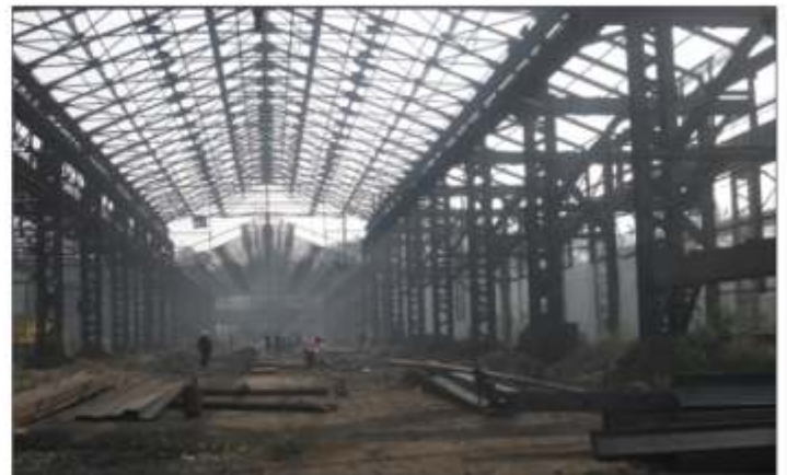
Work in progress at Wagon factory at Kulti, West Bengal
