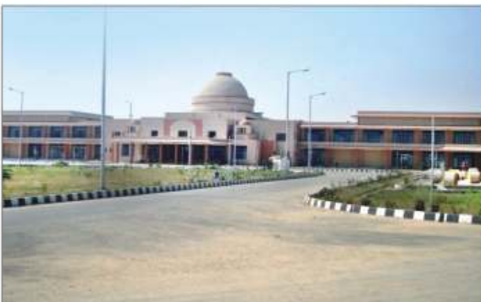
Planning Designing and Project Management of Integrated Check-post at Attari, Indo-Pakistan Border
