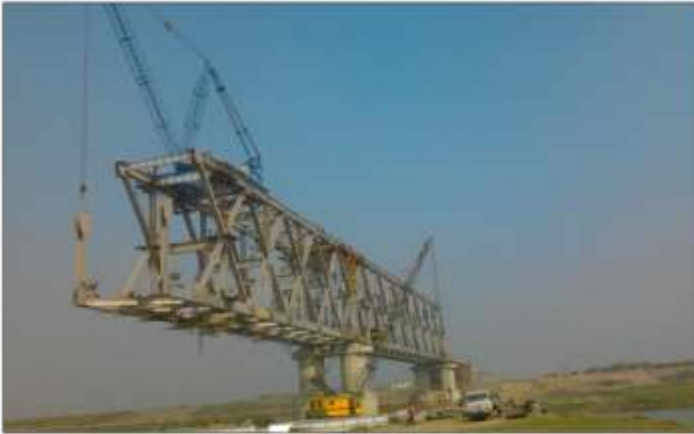
Rail-cum road bridge across river Ganga, Patna
