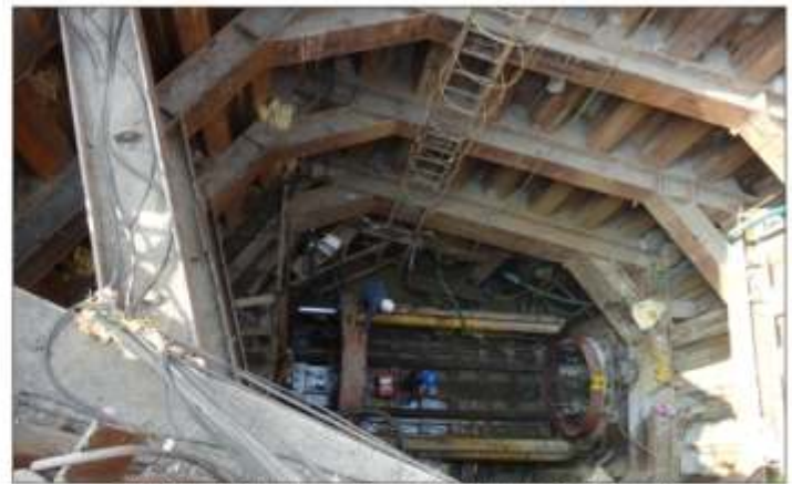
Tallah-Palta dedicated transmission mains for Kolkata Municipal Corporation
