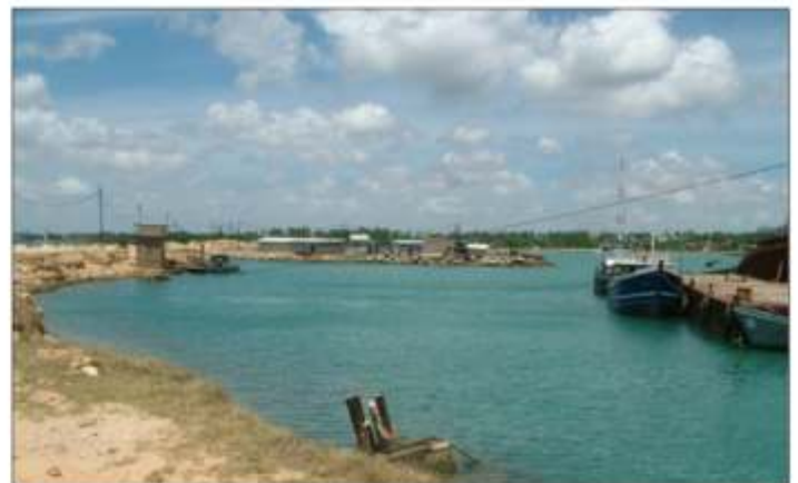
Detailed project report for rehabilitation of Kanakesanturai Harbour, Sri Lanka
