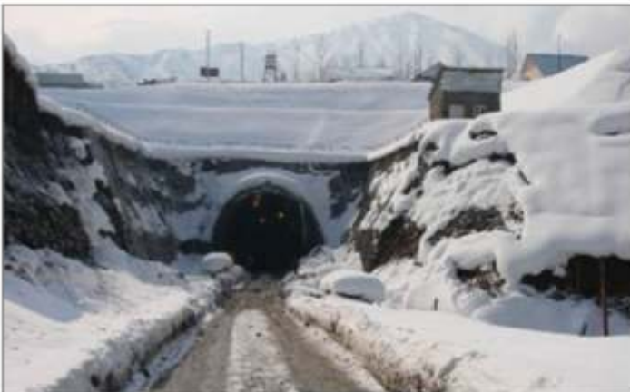
Pir Panjal Tunnel near Banihal, J & K
