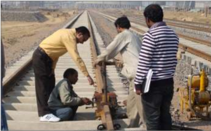
Trade linking works at Dadri
