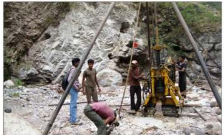
Geo-technical investigation in progress at site
