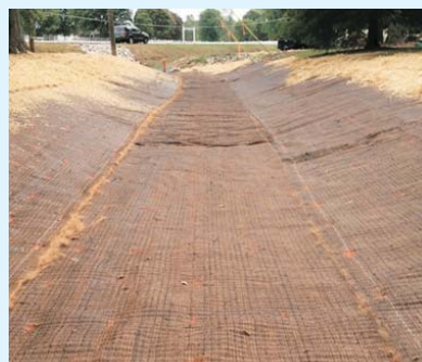
Road Construction with Buildtextile
