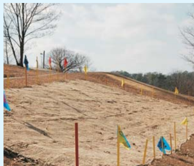
Slope stabilization with Geotextile
