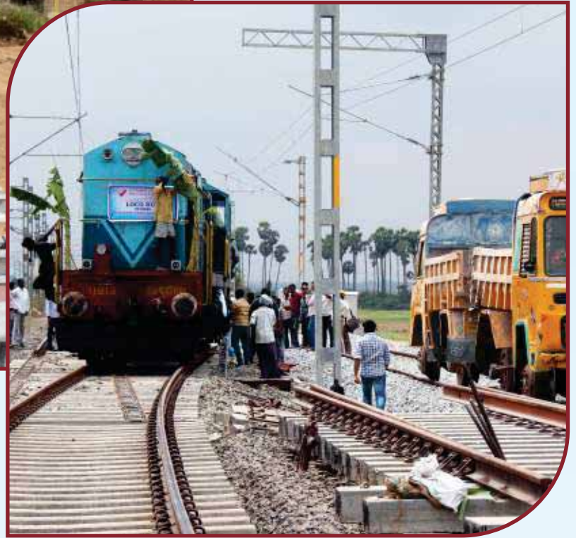
Loco Trial at Tiruvallur-Arakkonam 4th Line Project
