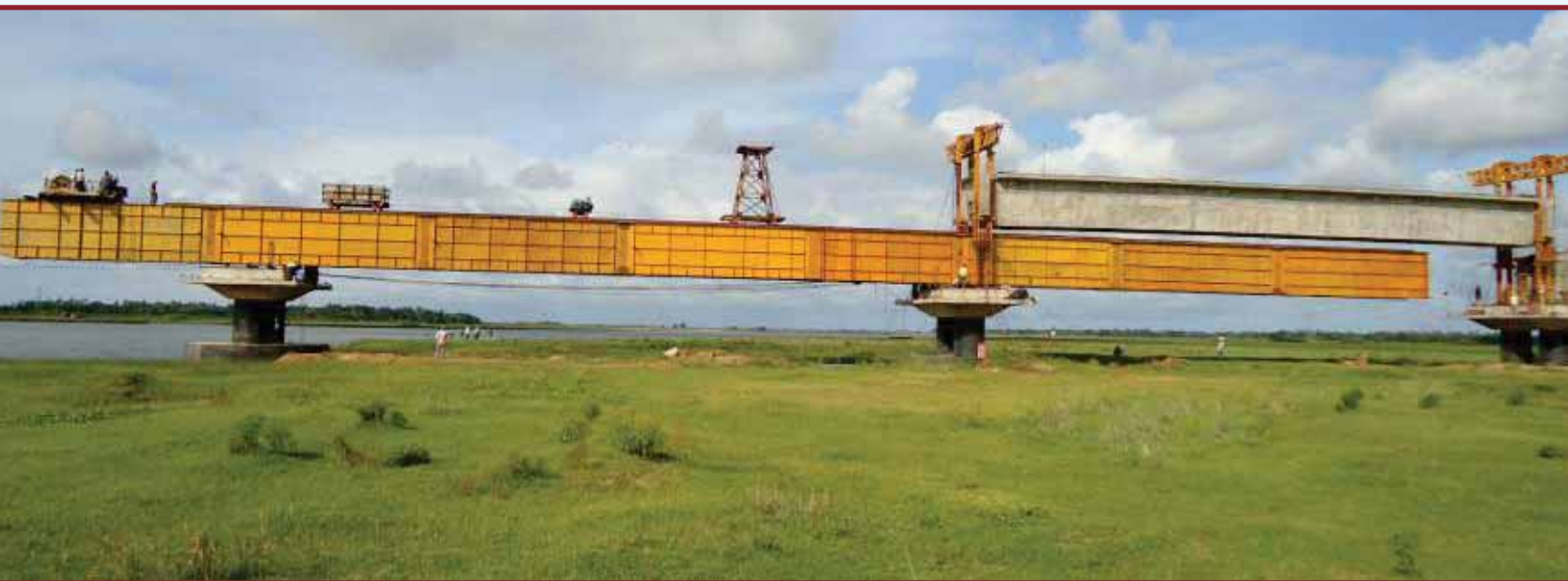
Bridge No. 134 on River Mahanadi in Haridaspur Paradip New Line Project
