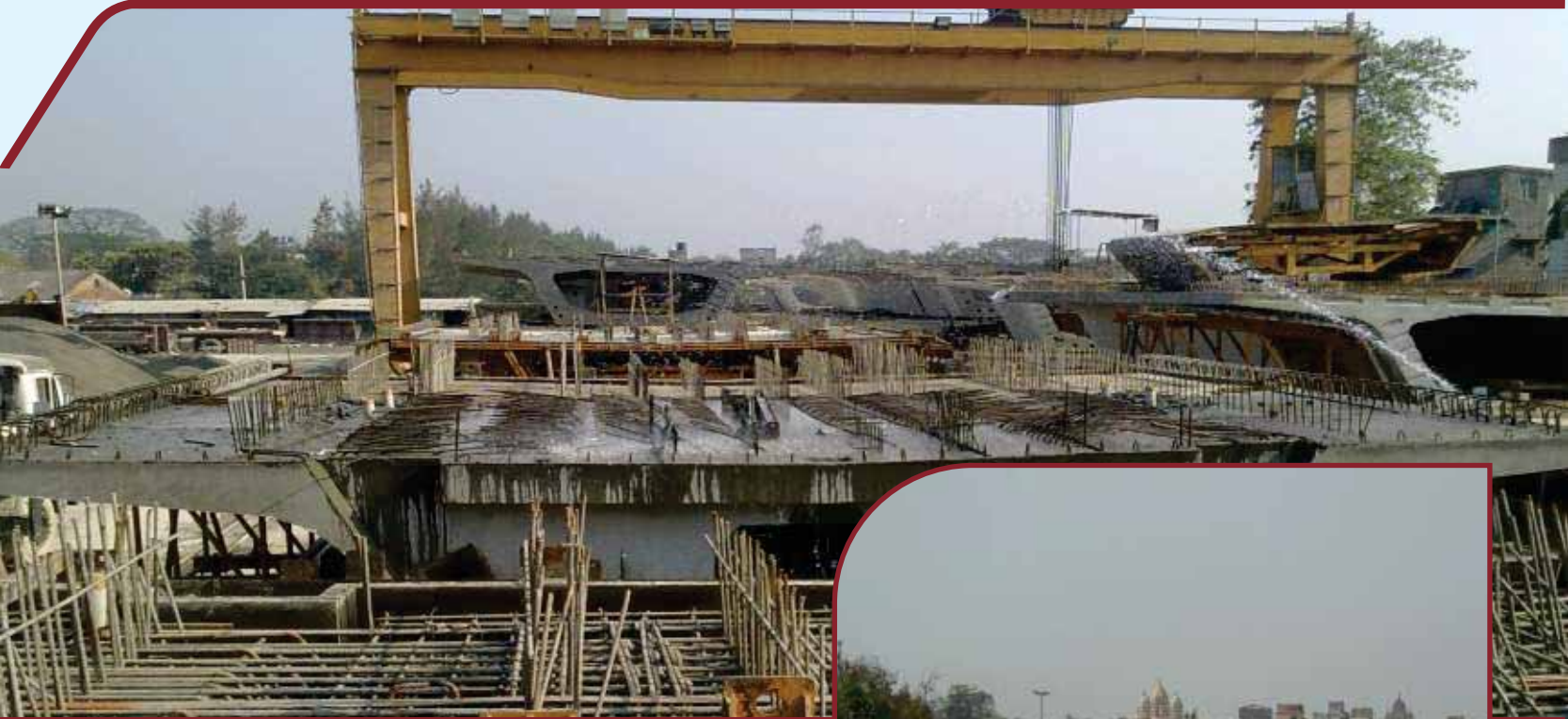
Joka BBD Bagh Metro Project, Kolkata
