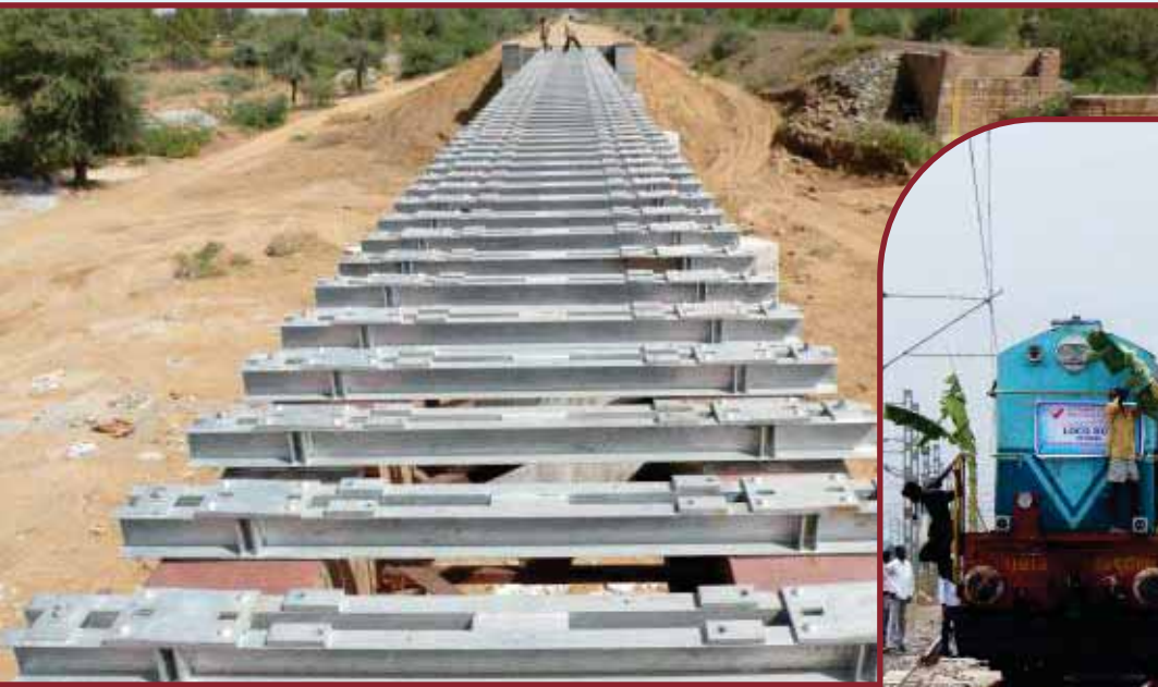
Bhildhi Samdhari Gauge Conversion Project
