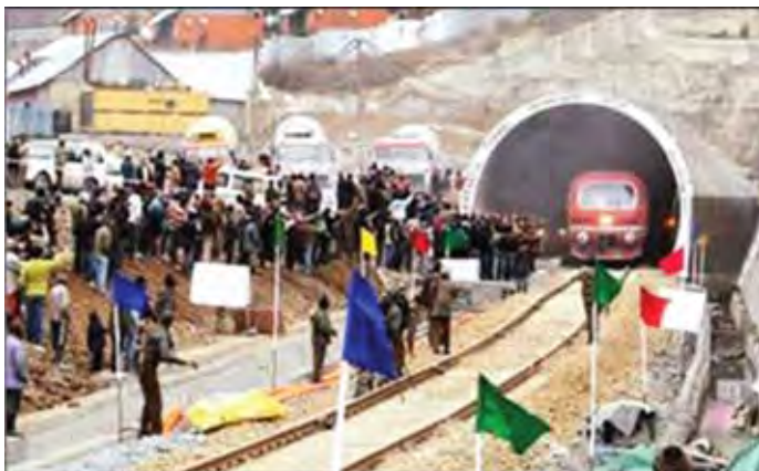
Detailed Design and Construction Supervision works for 11km long prestigious Pir Panjal Railway Tunnel and Northern Railway Tunnel No.1
