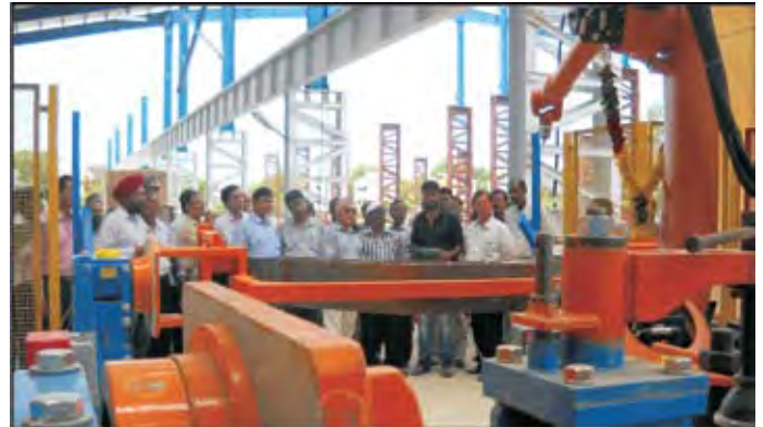
Turnkey work for FIAT Bogie Shop at ICF, Chennai: Installation of Robotic Welding machine
