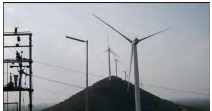
Wind Turbine, Thiruvavelli, TN
