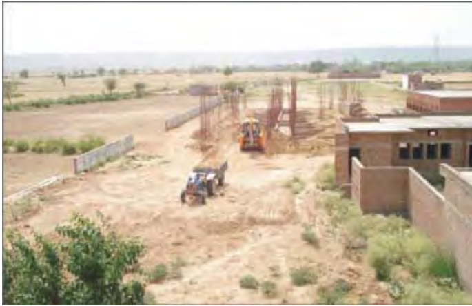
CSR: Construction of Girl's hostel at Khanpur Ghati, Mewat, Haryana
