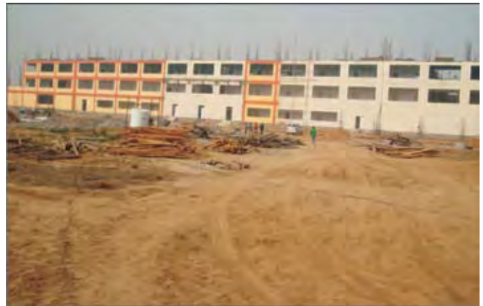
CSR: Construction of school complex at Village Wazirpur, Manesar
