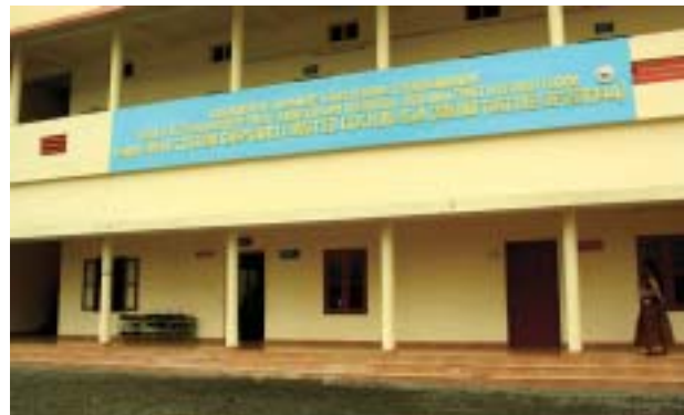
Financial support for building 1st & 2nd Floor of Saraswathy Vidhyanikethan High School, Chengamanad, Ernakulam.
