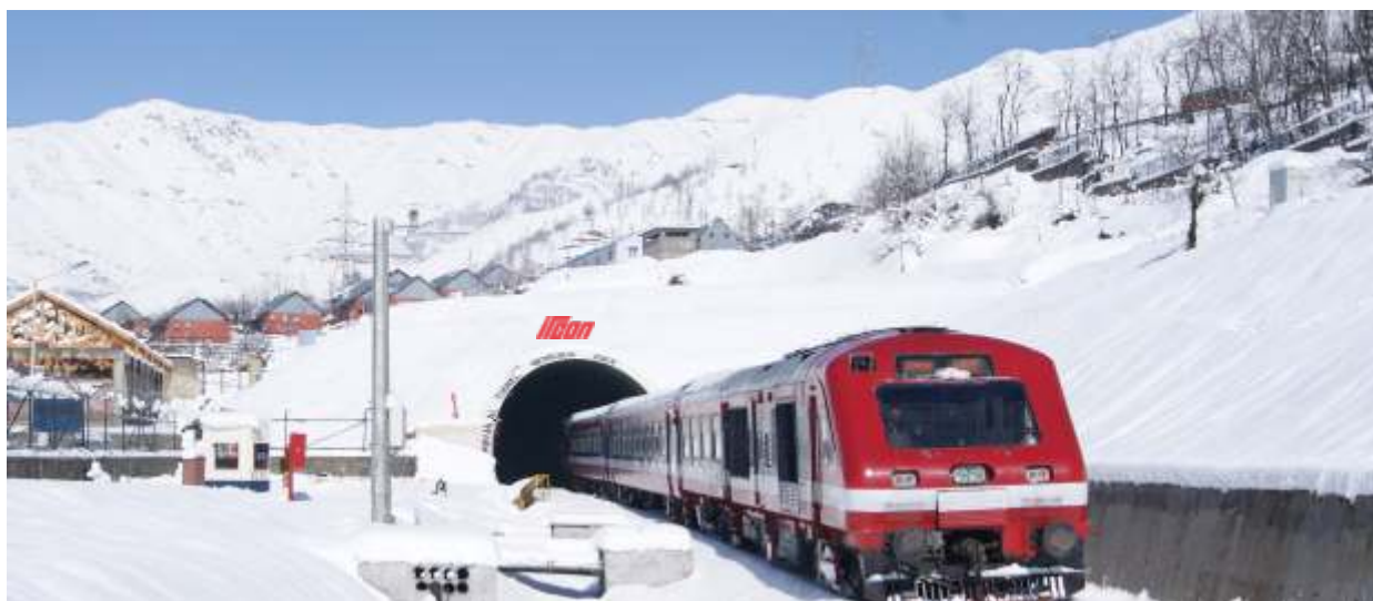
Train passing through 11 kms Pir Panjal Tunnel in J&K
