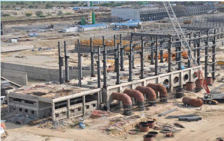
Cooling Water Pump House work at YTPS, Raichur
