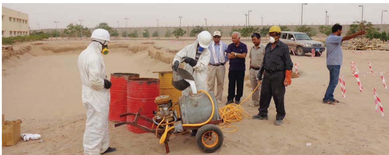
Anti-termite treatment at Yemen site
