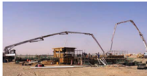
Casting of GT #5 at Yemen
