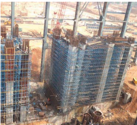
Turbine Generator Deck (TG Deck) staging arrangement at HNPIL, Vizag
