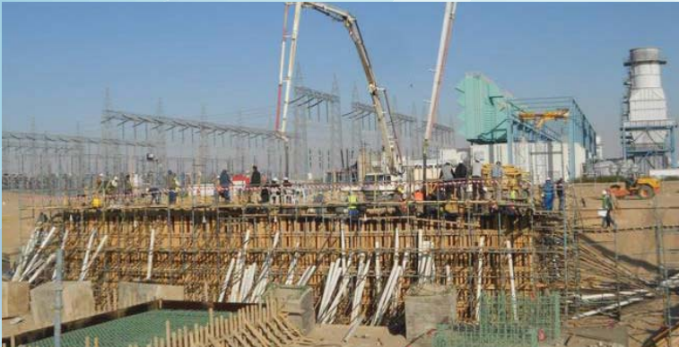
Casting of Gas Turbine #7 at Yemen
