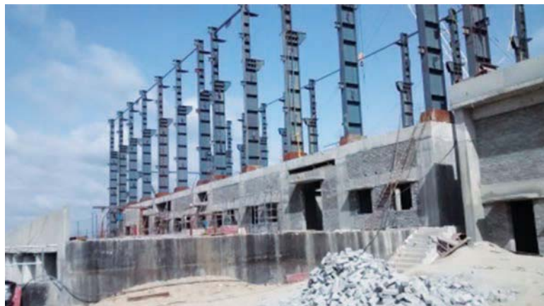
Cooling Water Pump House work at YTPS, Raichur
