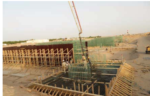
Casting of GT #7 at Yemen
