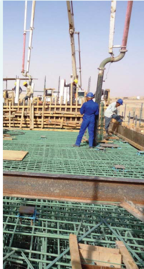
Casting of Gas Turbine #6 at Yemen
