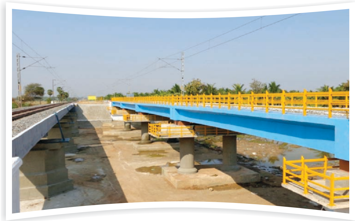
PSC Girder Bridge in Villupuram - Dindigul doubling project.
