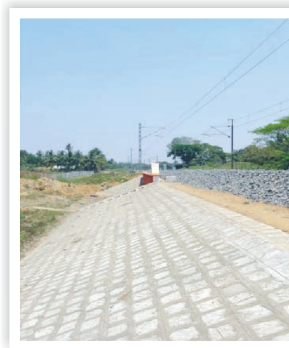
Stone Pitching at bridge approaching Villupuram - Dindigul doubling project
