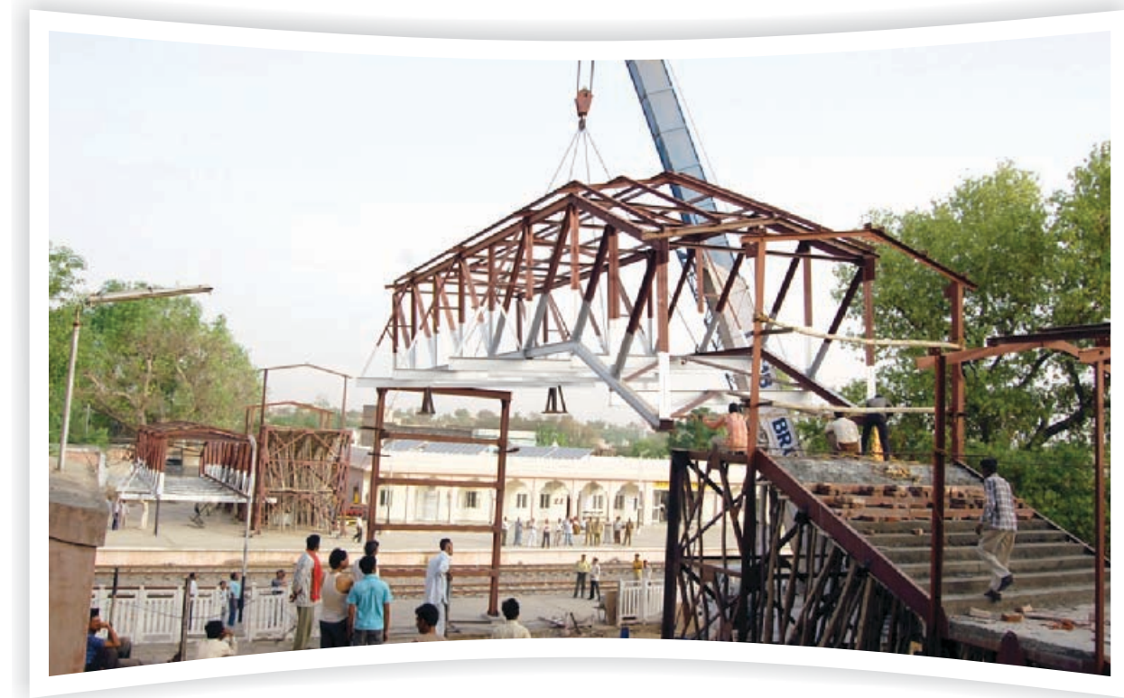
FOB launching at Nimka Thana - Ajmer - Phulera - Ringur - Rewari GC Project
