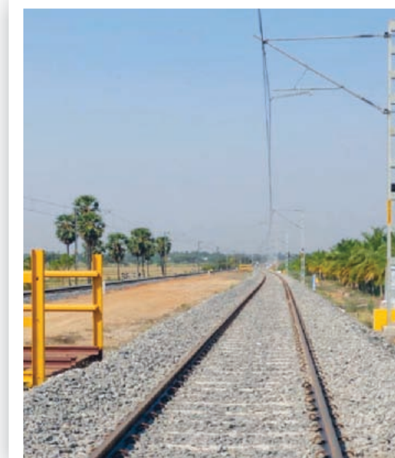
Machine Packed track of Tiruvallur Arakkonam line ready for commissioning
