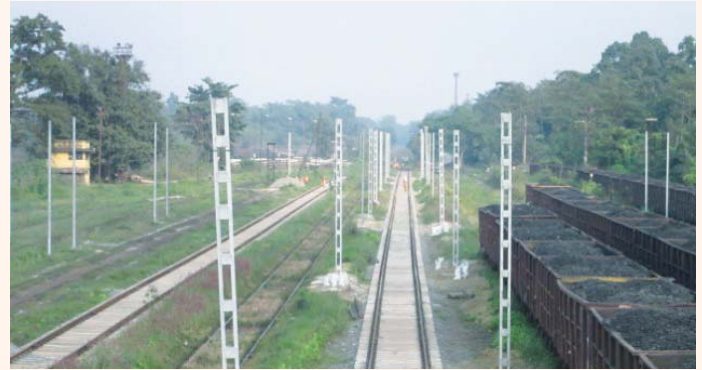
OHE works at SAIL Rourkela Plant
