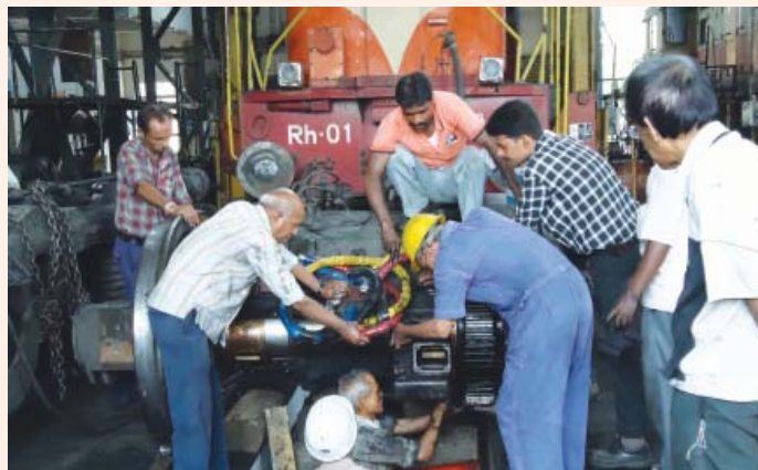
O&M of locomotives
