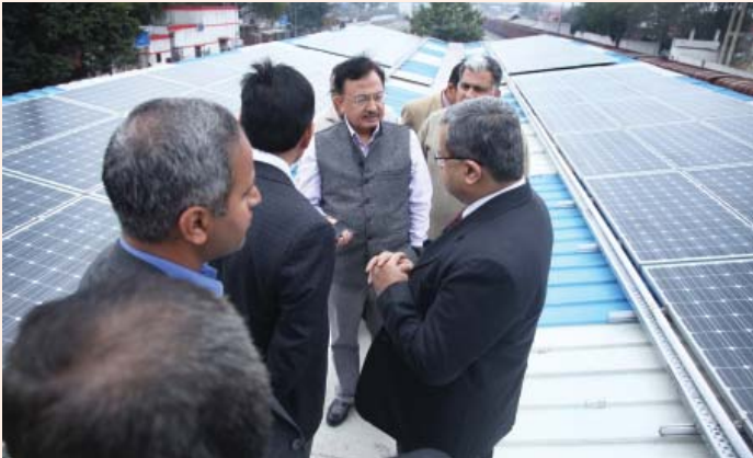
Inspection of the solar power plant at Gurgaon Railway station by the then General Manager - Northern Railway and CMD-RITES
