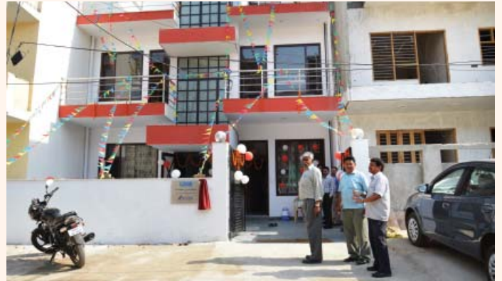
CSR: Youth Facility House for SOS Children’s Village Near Anangpur Village, Faridabad
