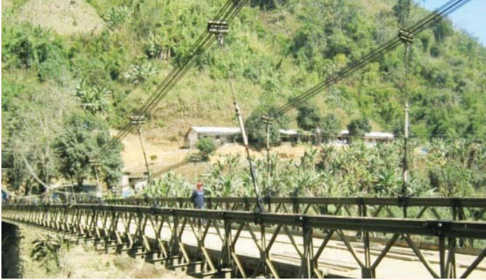
Bridge on River Barak in Manipur
