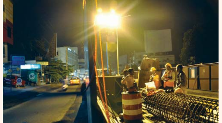
PMC for Kochi Metro Construction work at site
