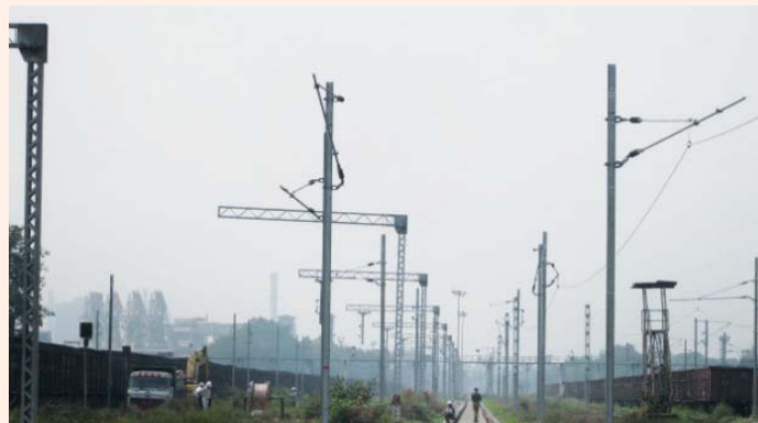
OHE works at SAIL Rourkela Plant
