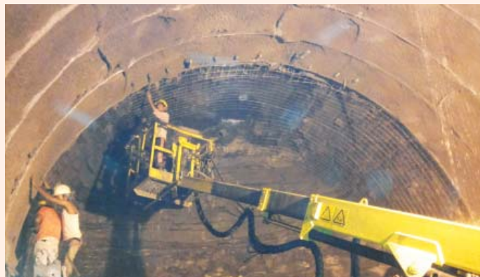
T10 Manipur Jiribaum Tupul Tunnel Work in Progress
