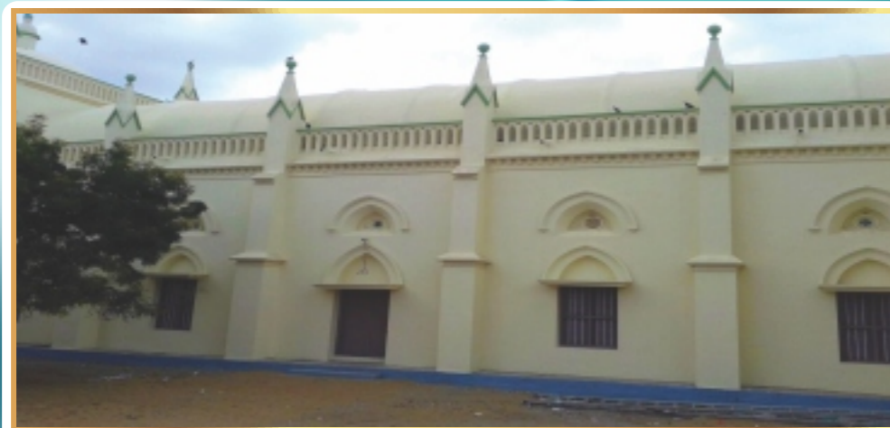
Church Roof Exterior(QuikBuild)-Vember
