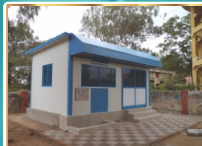
R.O unit at Hindupur, AP (ISO BUILD)
