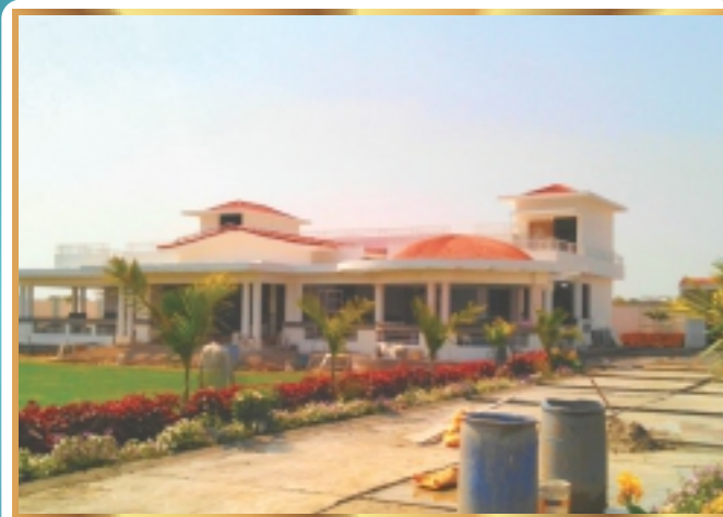
Farm House (QuikBuild) - Hyderabad
