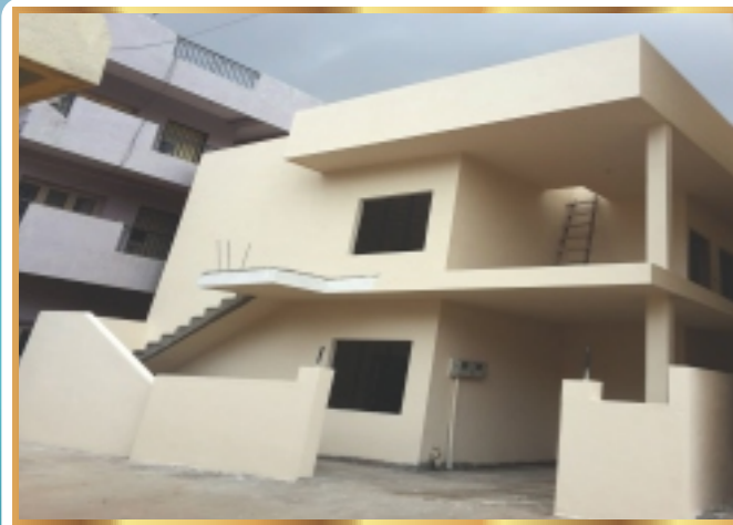
G+1 House at Marathahalli (QuikBuild) - Bangalore
