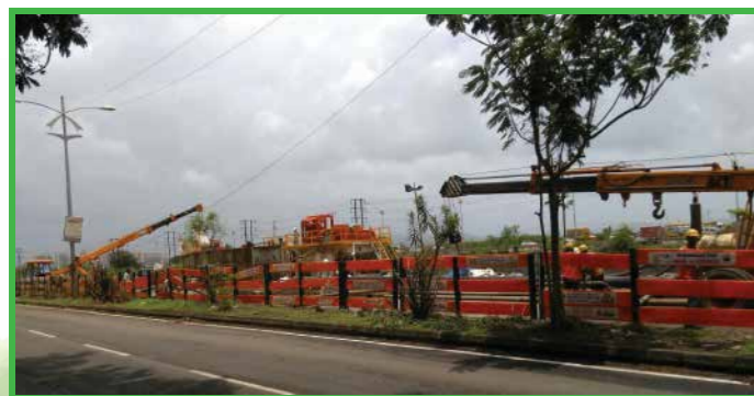
Kharghar Creek pipeline laying site.
