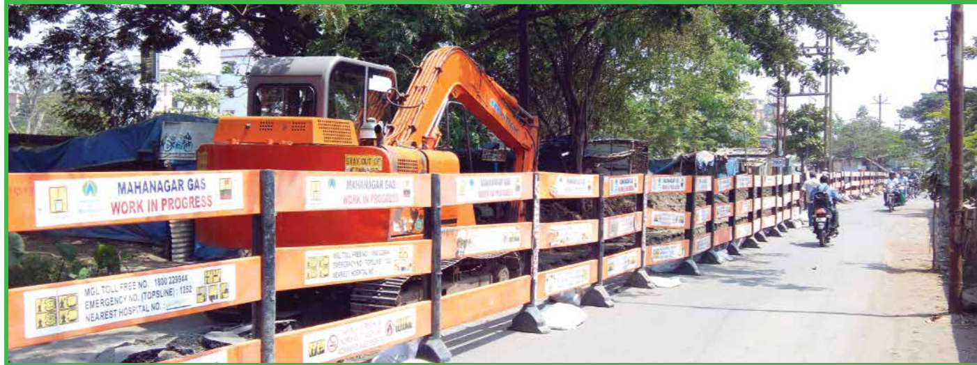
MGL steel pipeline laying site.
