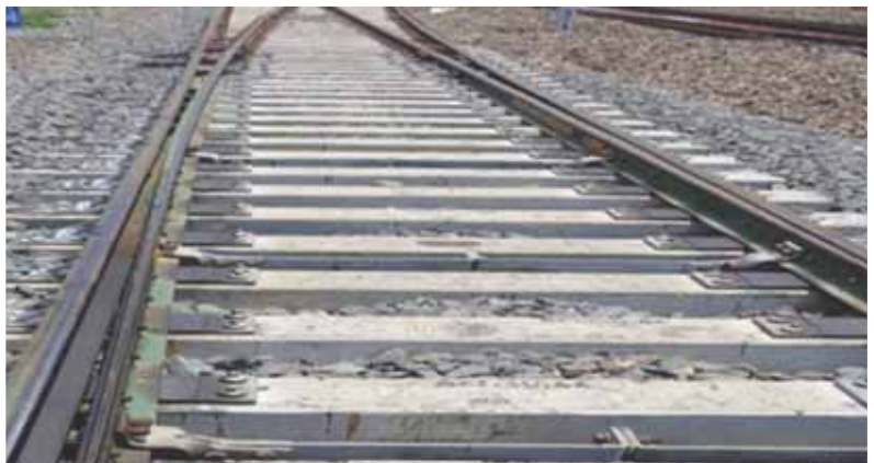
Galvanised Track Fittings on Points and Crossings
