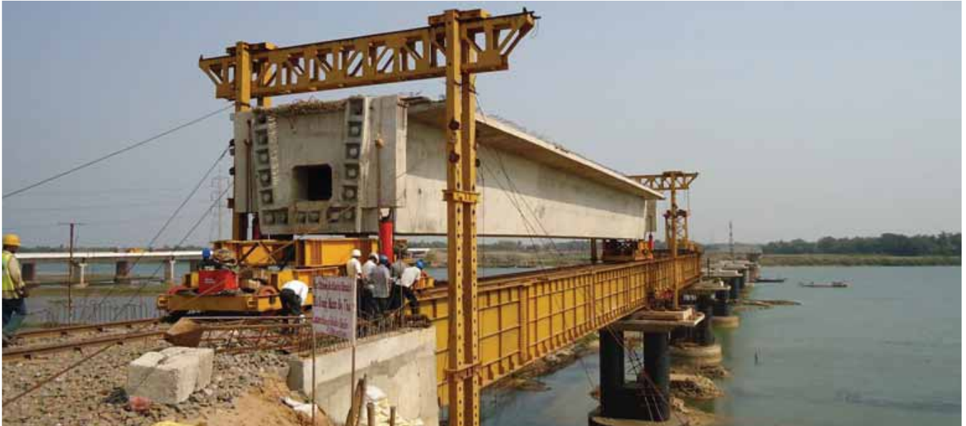
PSC Girder on Luna Bridge
