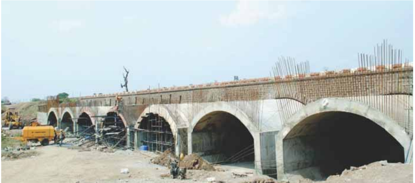
RCC Arch Top Box for the doubling line
