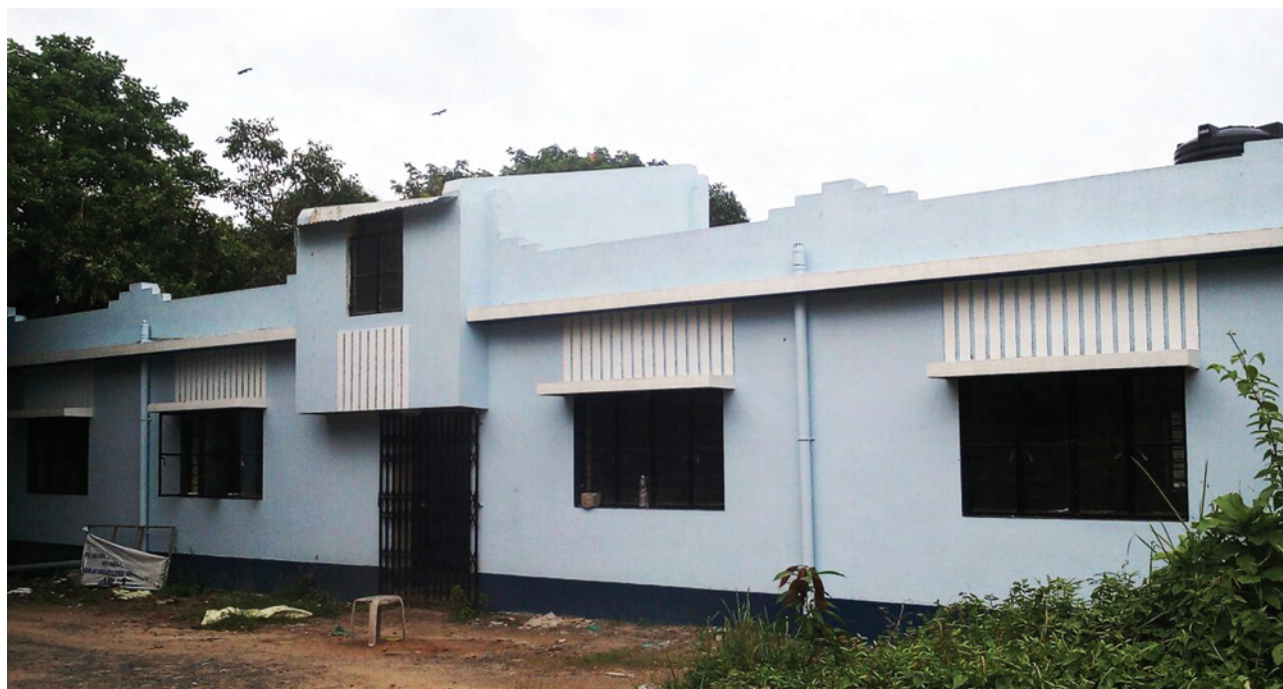
Night Shelter at Kolkata under HUDCO - CSR Activities
