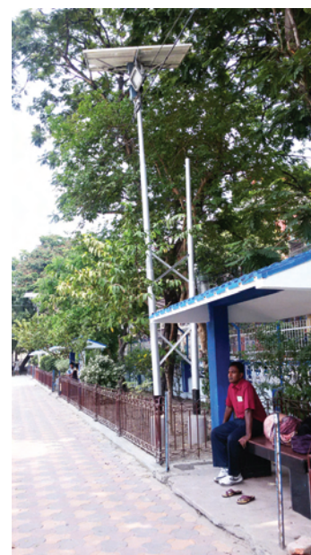
Solar Lighting at Deshapriya Park, Kolkata
