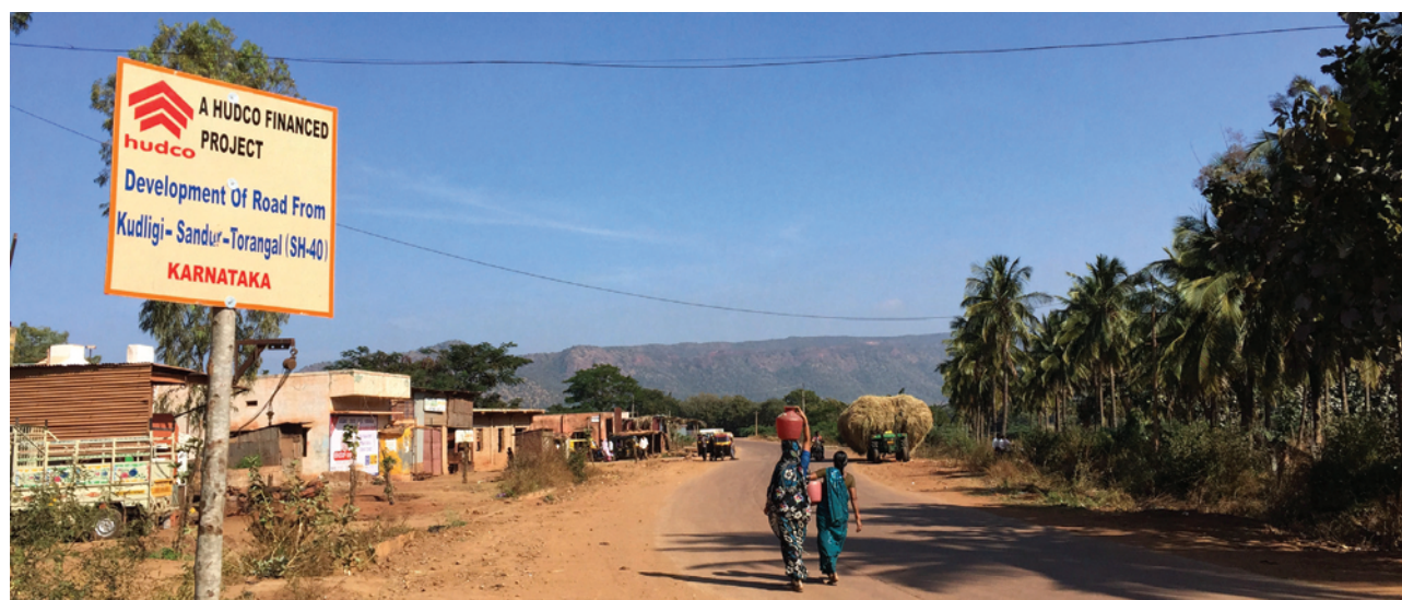
HUDCO financed road project at Bellary, Karnataka
