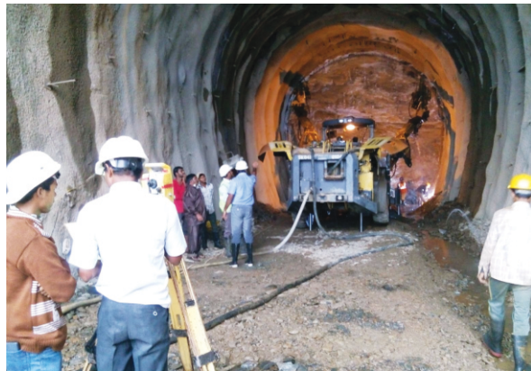
Tunnel work being executed by PIU/Chennai
