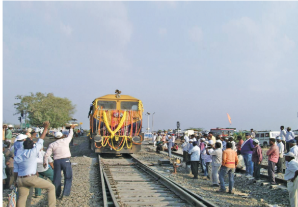
Opening of New UP Main Line between Hotgi & Tilati (New) Section of Solapur Division, Central Railway
