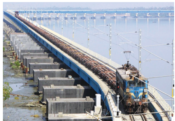
Container Train on Vembanad Bridge Cochin
