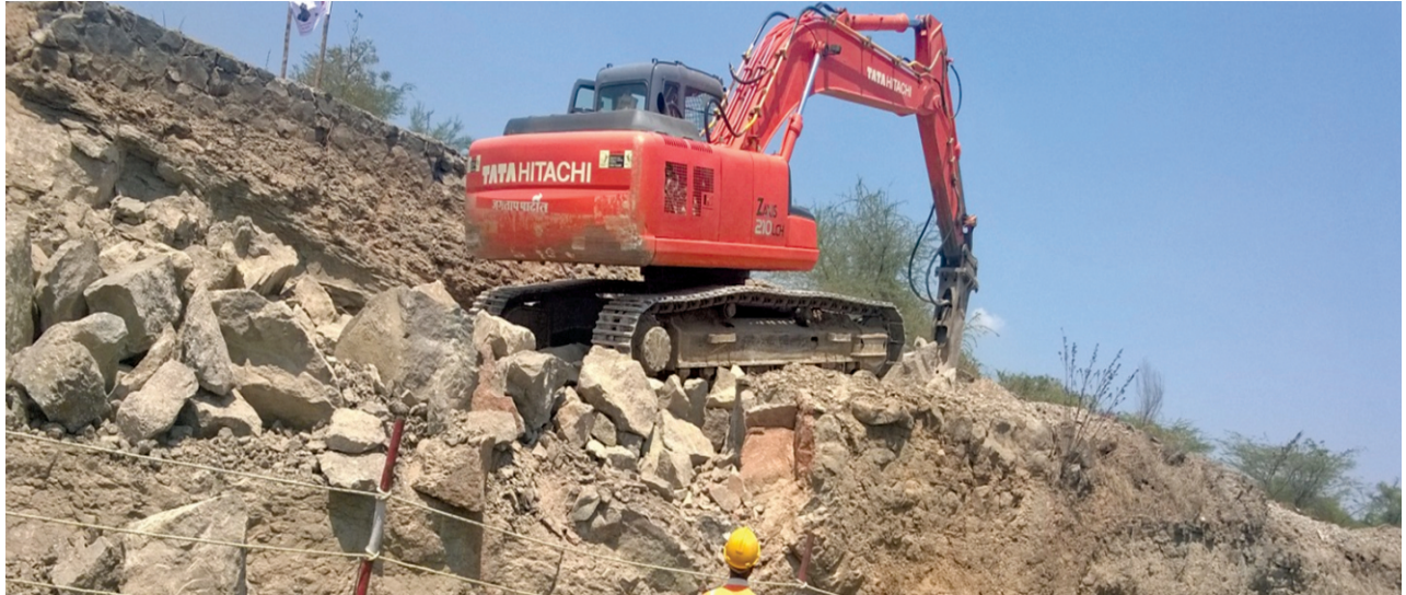
Cutting work in Progress at Km 304-305
