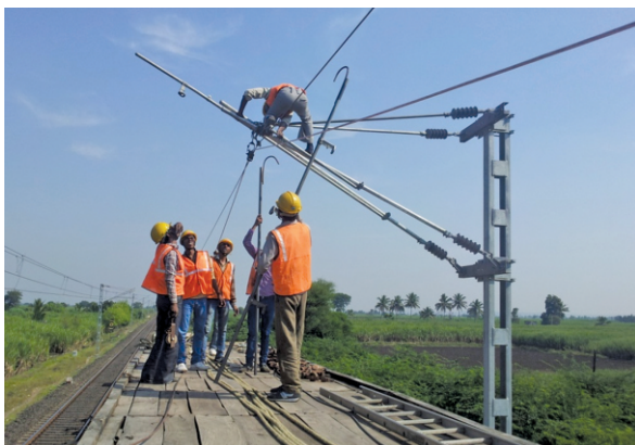
OHE wiring works in Daund-Patas Section (72 RKM)
