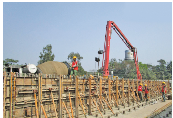
Casting of I-Girder at Casting Yard
