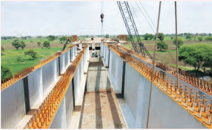
Project Management Consultancy Services for Cable Stayed Bridge - Nagpur
