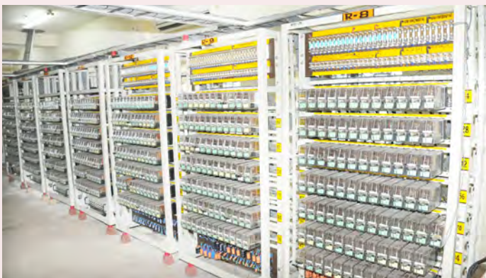
Railway Electrification work at Rourkela Steel Plant Railway Siding
