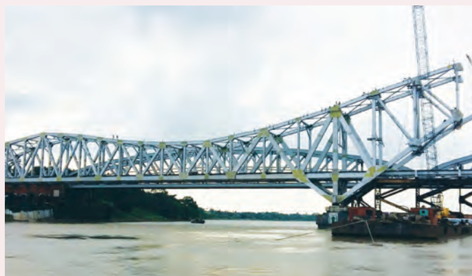
Jubilee bridge under construction
