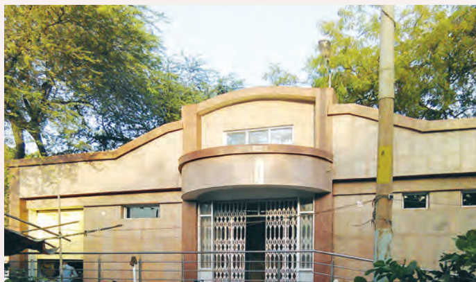
Public Toilet Complex at Gurgaon Railway Station, Haryana
