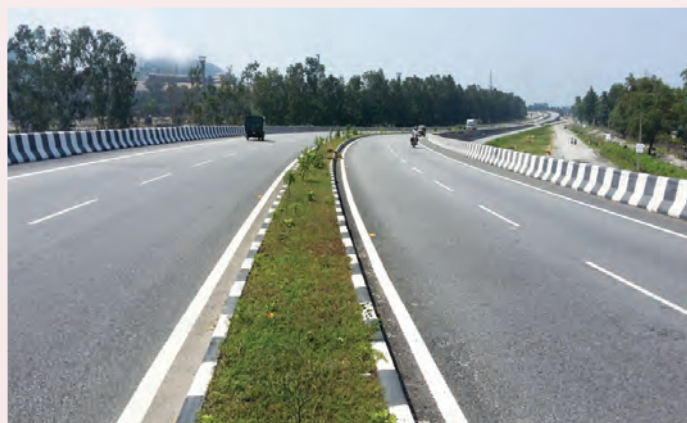
Four-laning National Highways works, Assam
