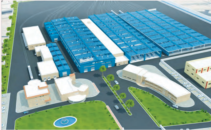
Gyaspur metro depot at Ahmedabad
