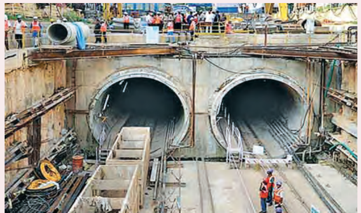
Tunneling work in progress- Delhi metro
