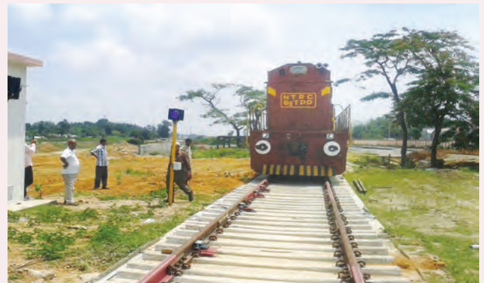
Weigh Bridge at NTPC
