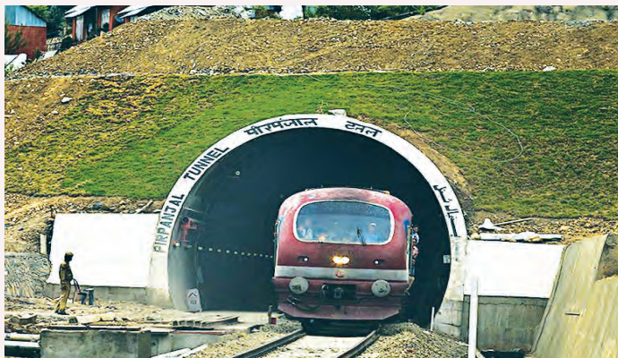
Pir Panjal Tunnel, Kashmir
