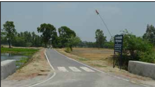
Bitumenous Road constructed at Barauliya, Korwa
