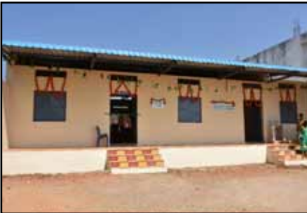
Kitchen, Dining Hall & Toilets Constructed at Janwada, Telangana
