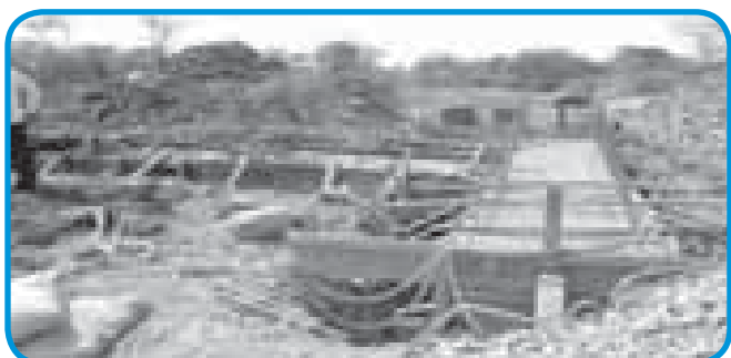
Cement Nala Bund (CNB) construction at Shelgaon, Pune
