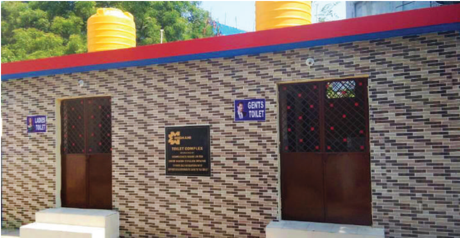
Toilets constructed by MIDHANI under 'Swachh Bharat' initiative.
