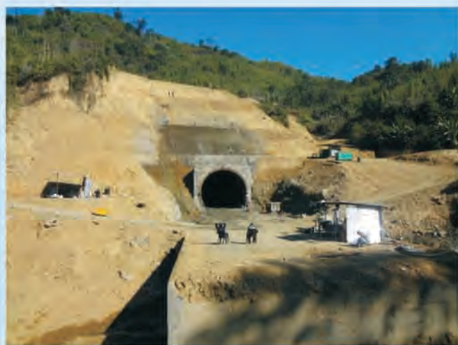
Construction of Portal of Tunnel - T11
