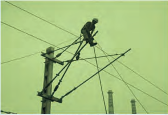
RE Siding work for SAIL, Rourkela Steel Plant
