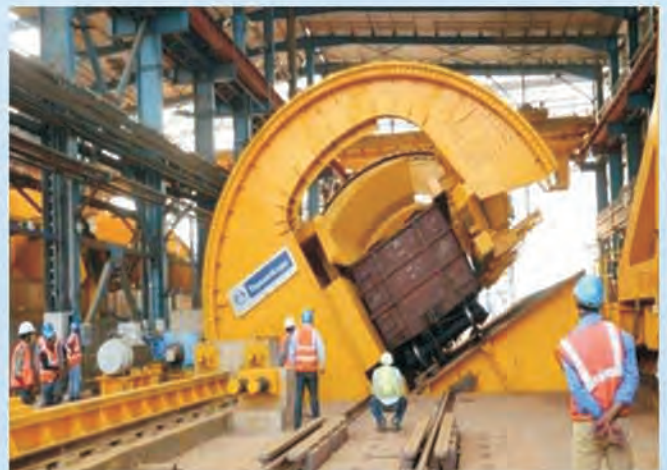
Unloading by Wagon Tippler at Tata Steel Ltd., Kalinganagar
