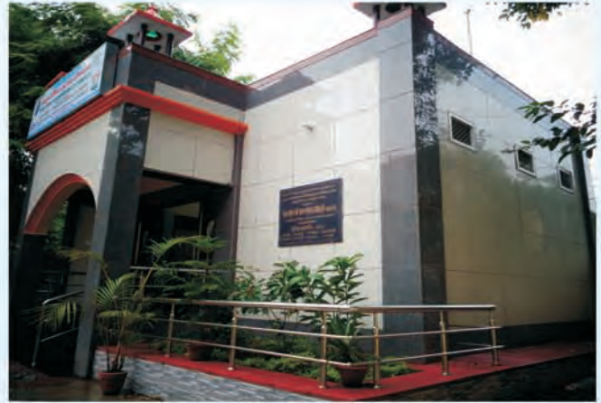
Public Toilet Complex in Varanasi, U.P., under RITES CSR
