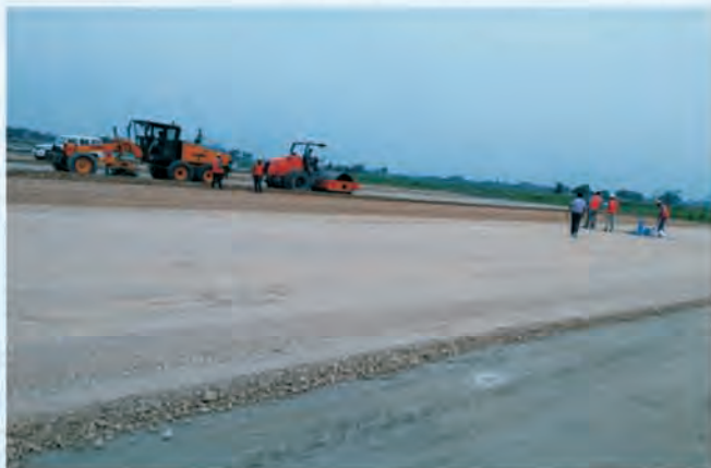
Sub Grade MDD Testing at Apron area
