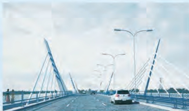
Proposed State-of-Art Extra-dosed cable stayed bridge over river Ganga in West Bengal
