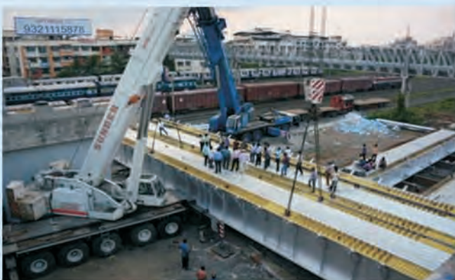
Launching of 24 M Girder at Vasai ROB under supervision of RITES
