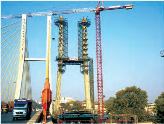
Cable stayed bridge at Santra Market, Nagpur
