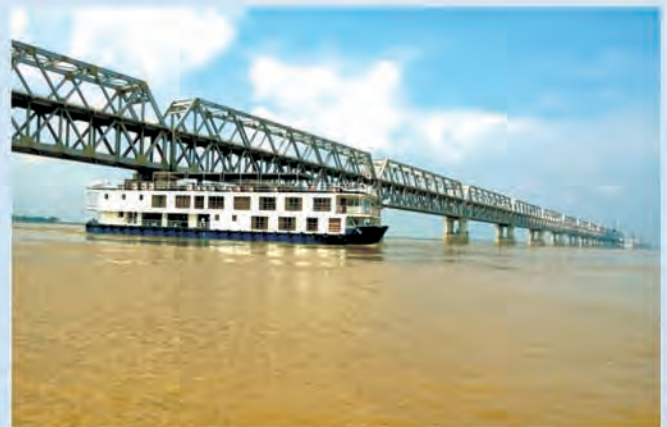
Recently completed 4.56 km Long Rail cum Road Bridge at Patna
