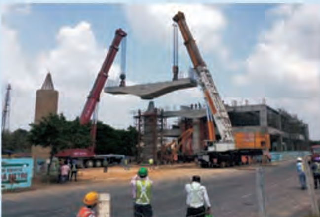
Launching of Precast pier cap in Noida, Greater-Noida Metro
