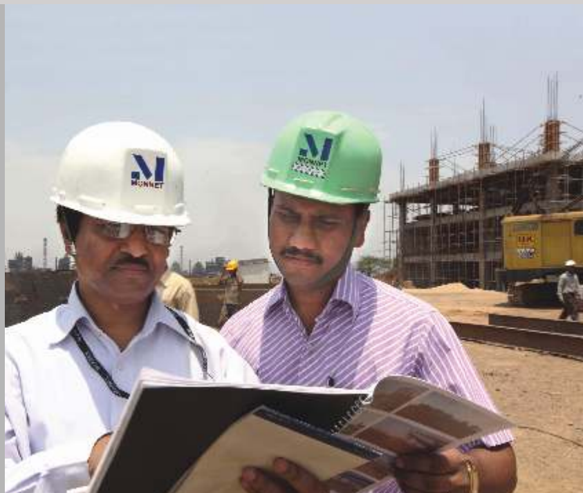
Expansion project at Raigarh in full swing
