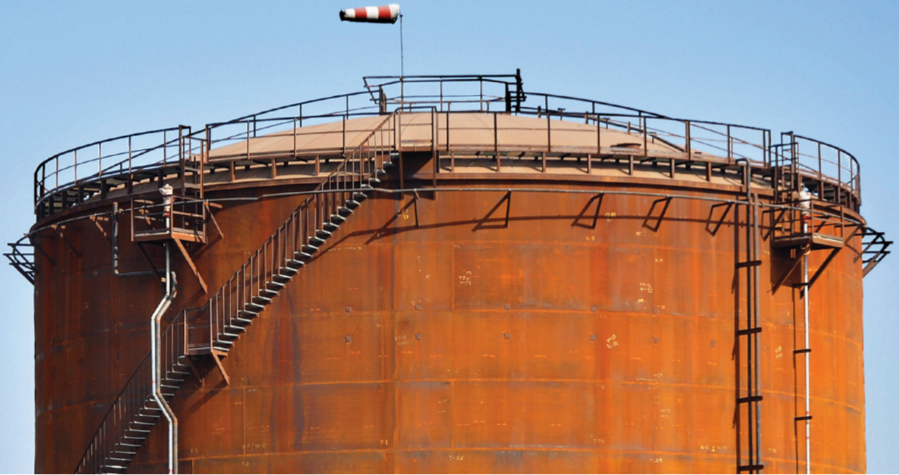
A tank under construction at the Pipavav terminal.
