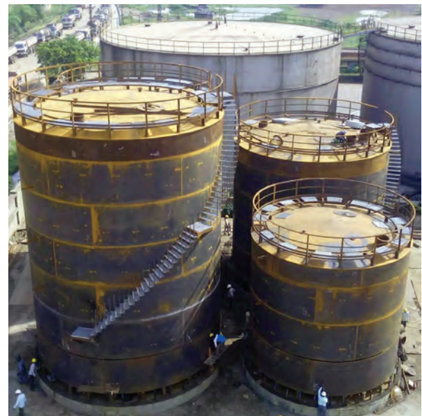
New liquid tanks under construction at Haldia
