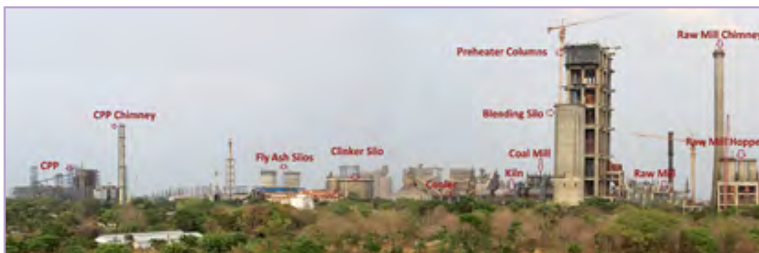
Wide angle eye-view of Manikgarh Cement Unit II with legend in red, 2.8 million tpa expansion unit (under construction) adjacent to the existing unit, Gadchandur, Dist. Chandrapur, Maharashtra
