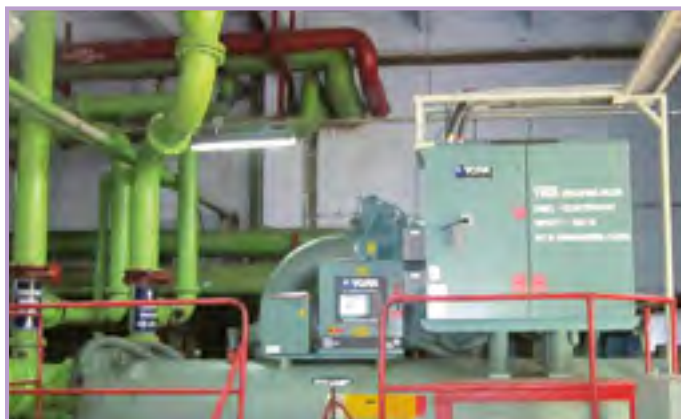
Eco-friendly energy efficient centrifugal chiller
