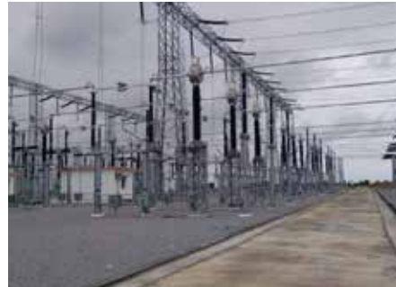
Commissioned 400KV CTS, GCBS and LA and 145KV CTS at Tstransco Narsapur s/s
