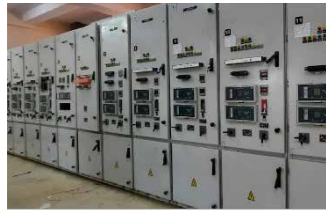
Commissioned 33 kv and 145 KV GIS at DMRC Charkop s/s at Mumbai
