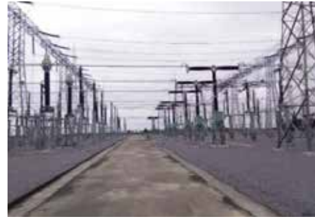
Commissioned 400KV CTS, GCBS and LA and 145KV CTS at Tstransco Narsapur s/s
