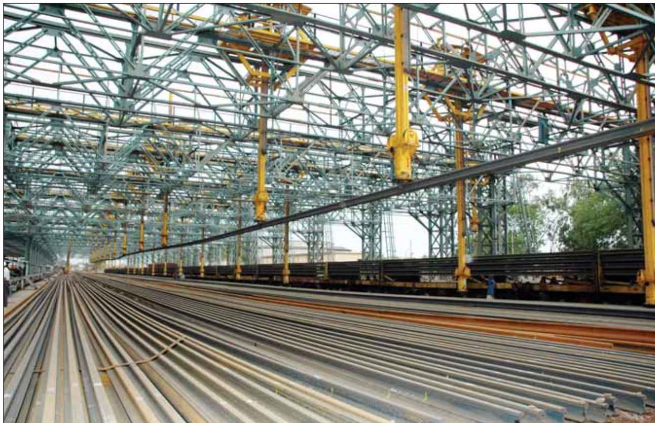
An overview of long rails at SAIL's Bhilai Steel Plant.
