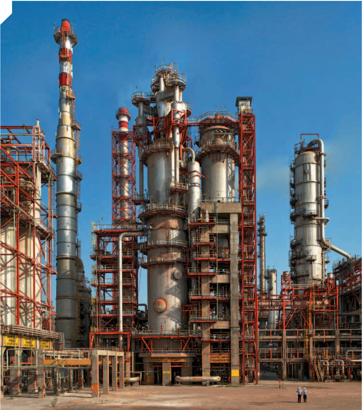
> FLUIDISED CATALYTIC CRACKING UNIT AT VADINAR
