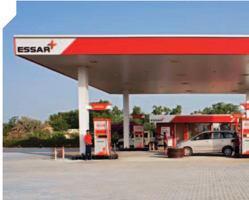
> ESSAR OIL RETAIL OUTLET AT BHUJ
